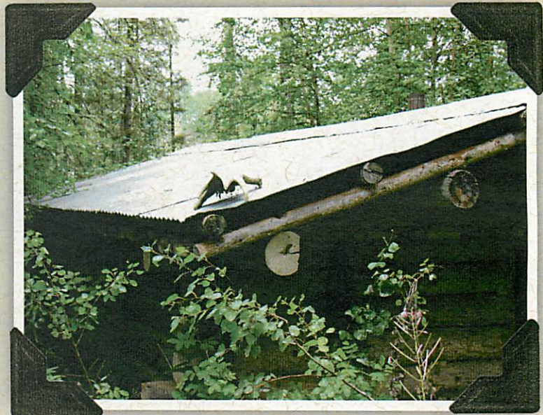
Photo #45: Crooked Lake Cabin Roof
