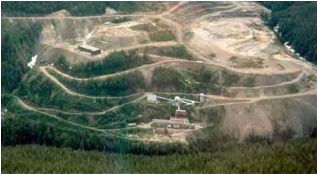
Figure 3.1-4: Mill Site Prior to Demolition
