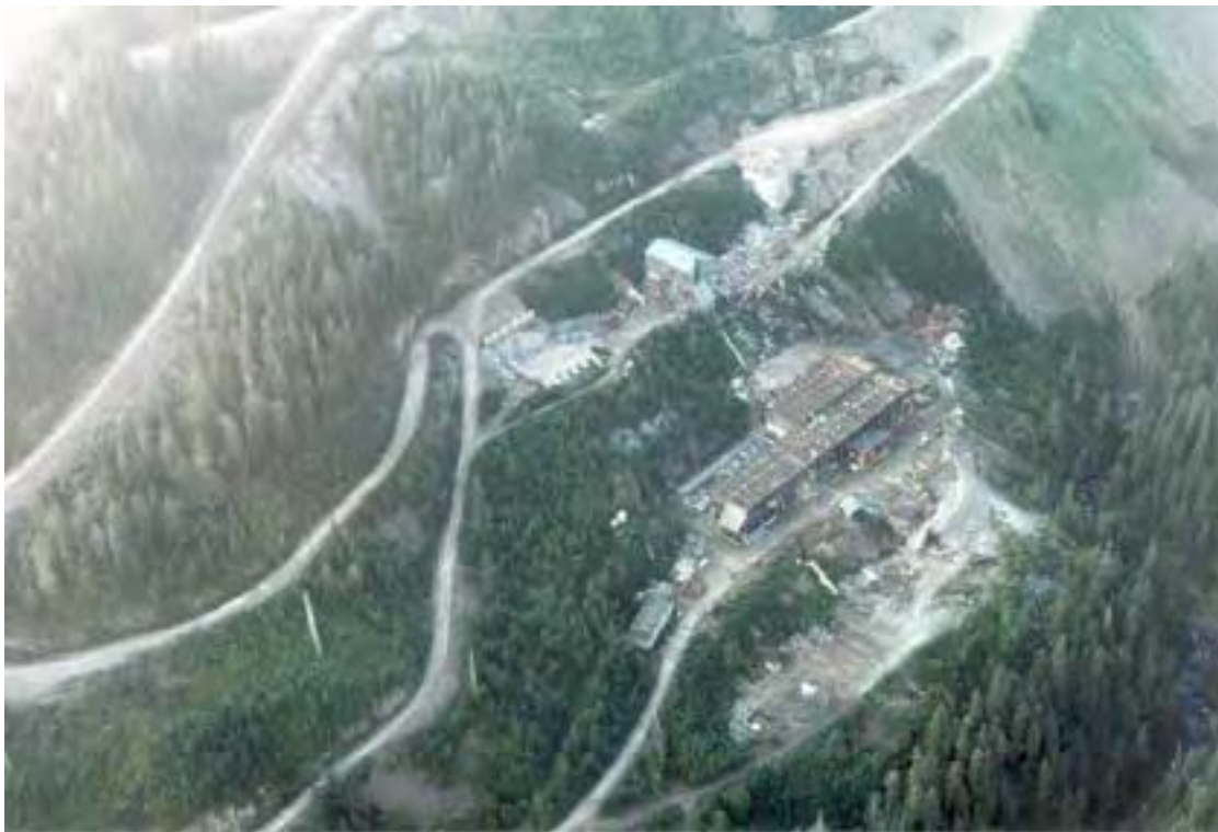
Figure 3.1-5: Mill Area During Demolition (1997)
