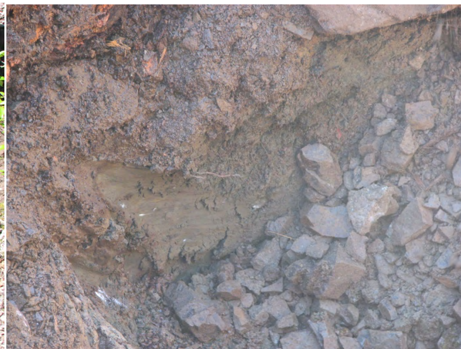
PHOTO 37 – TP10-01 silt deposit
