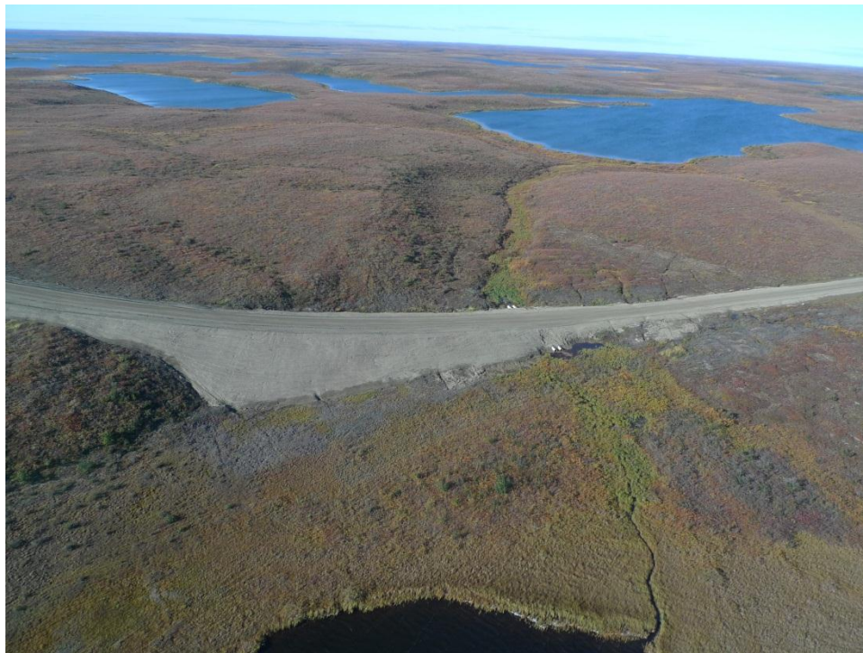
Source 177 Road showing a typical fill type construction method
