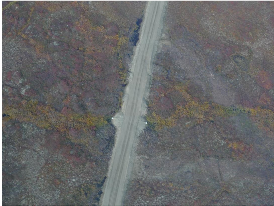
Source 177 Road showing a Drainage Culvert
