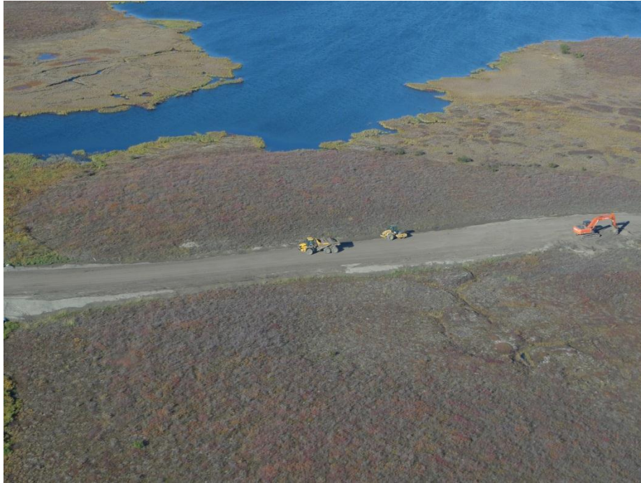
Construction/Maintenance Activities along Source 177 Road
