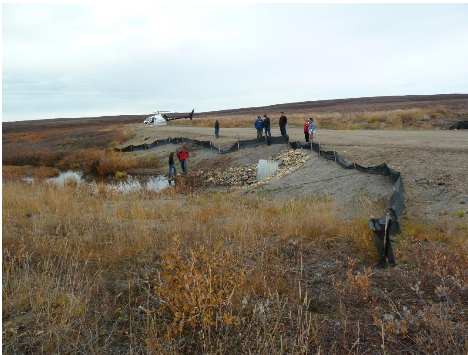
Source 177 Road Culvert Inspection by the Review Panel
