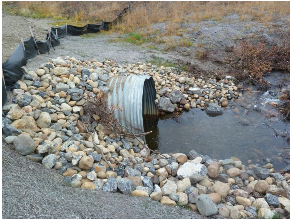
Source 177 Road close-up of one end of a Culvert
