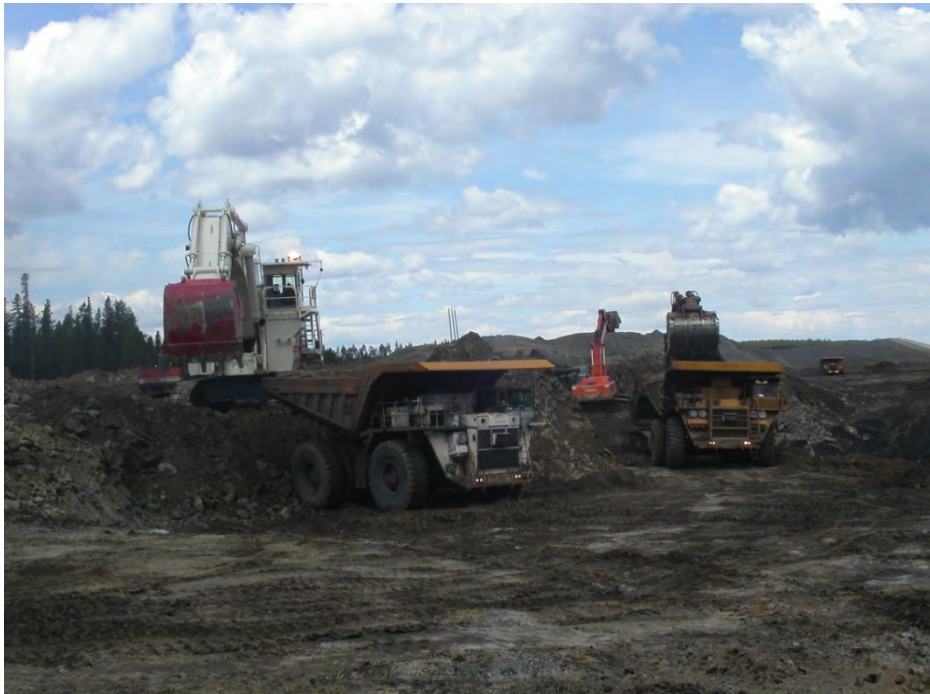
Figure 3 Large backhoes used to load haul trucks
