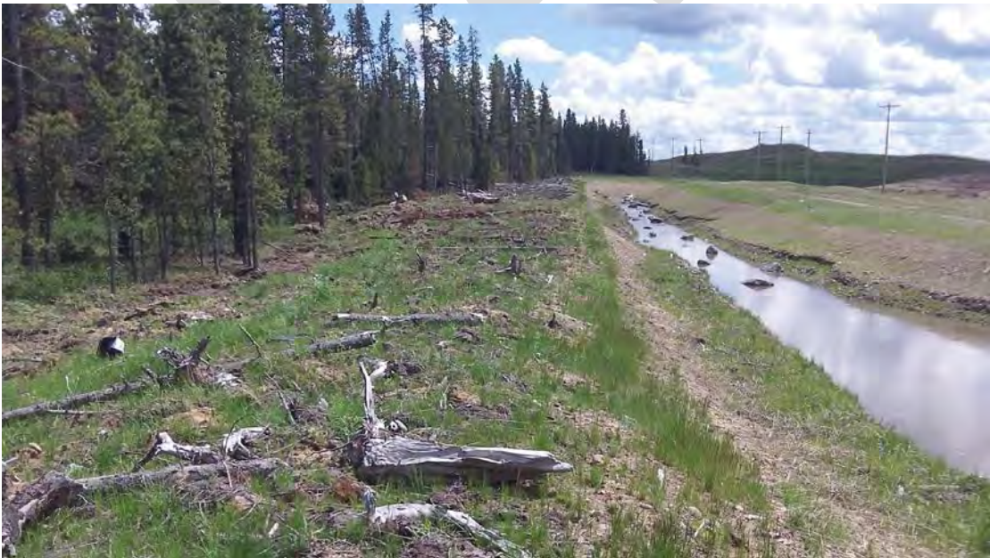
Looking upstream from Embarrass Exclusion Weir
