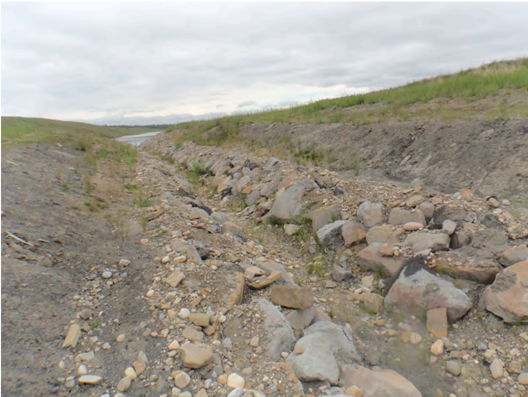
Figure 27. Existing channel between Pit 142W Lake and Upper Embarras Lake.
