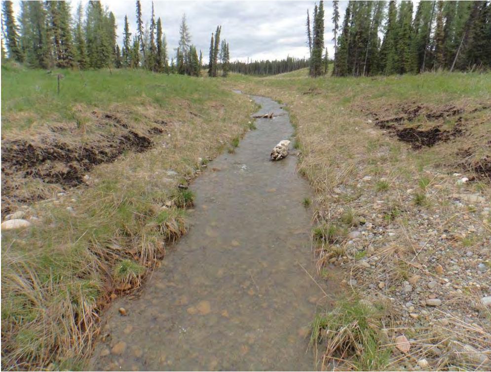
Figure 9. 25E Creek approximately 100 metres downstream of 25S Lake.
