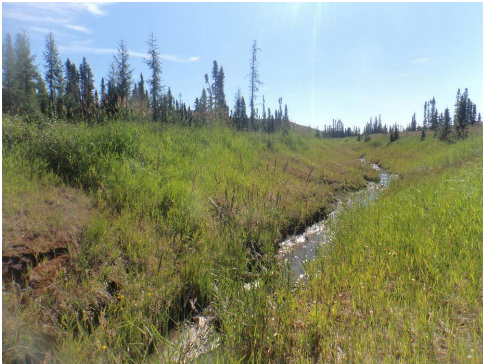
Photo 4. Looking upstream at representative stretch of the Mercoal Diversion.
