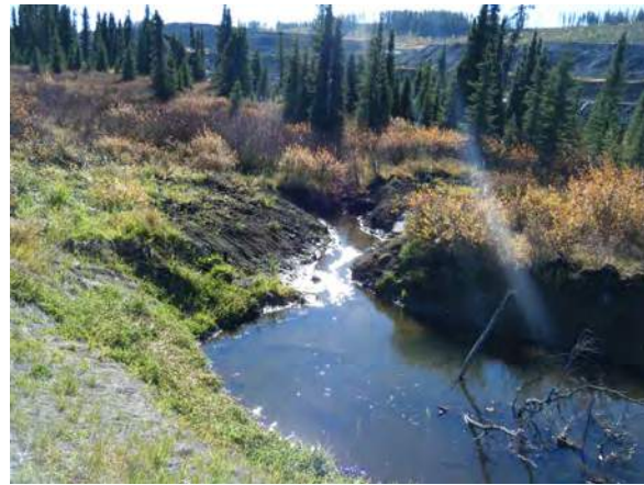
Photo 4. Looking u/s at the u/s tie-in of the diversion channel.
