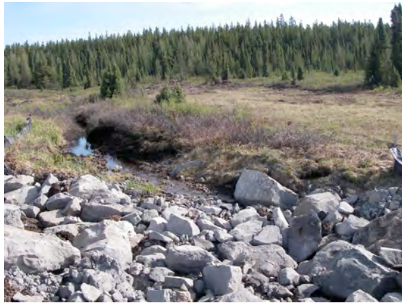
Photo 1. Looking upstream at MET-3 channel from upstream end of restored channel.
