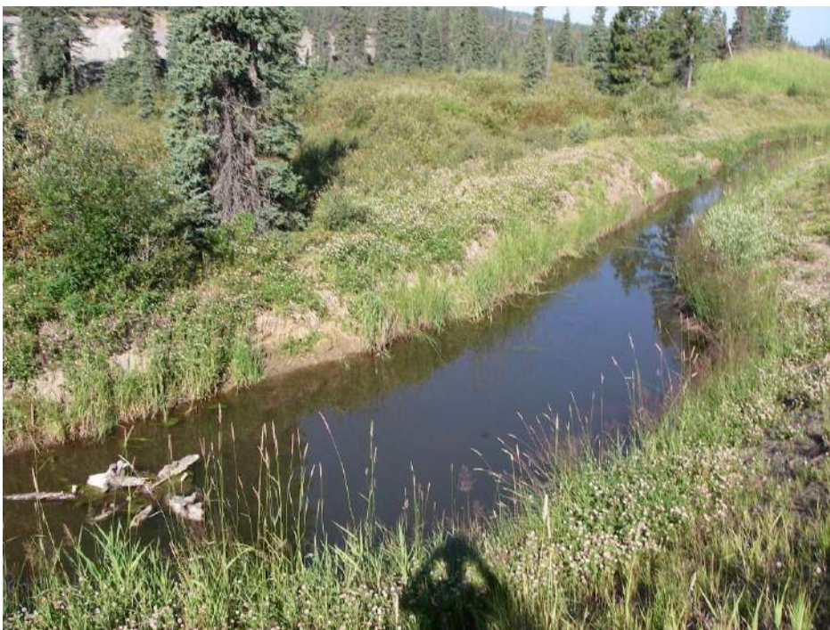
Figure 11. Upper Mercoal Creek diversion channel in summer 2012.
