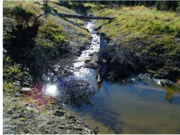
Photo 2. Looking u/s at an anchored tree within the diversion channel ~260 m u/s of the d/s end of the dc.
