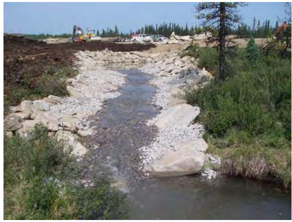
Photo 14. Looking upstream at outlet channel from downstream tie-in.
