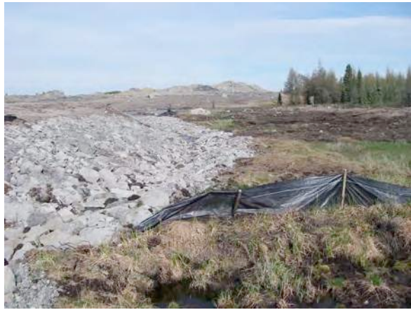
Photo 3. MET-3 Restored channel overview (looking downstream).
