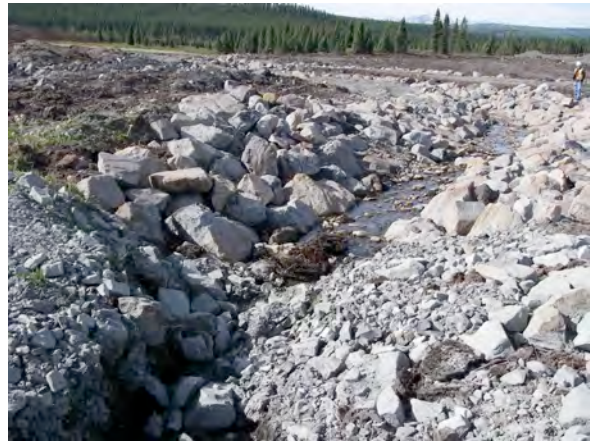
Photo 4. MET-3 Restored channel where surface connectivity resumes (looking downstream).
