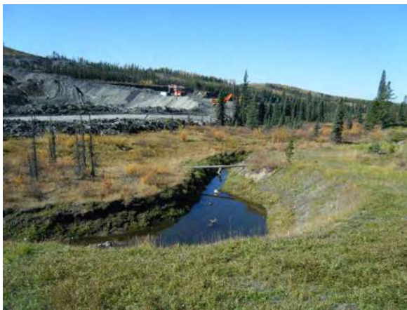
Photo 5. Looking downstream from near the u/s end of the diversion channel.
