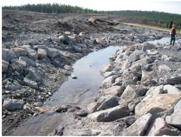
Photo 5. Looking downstream at lower restored MET-3 channel.
