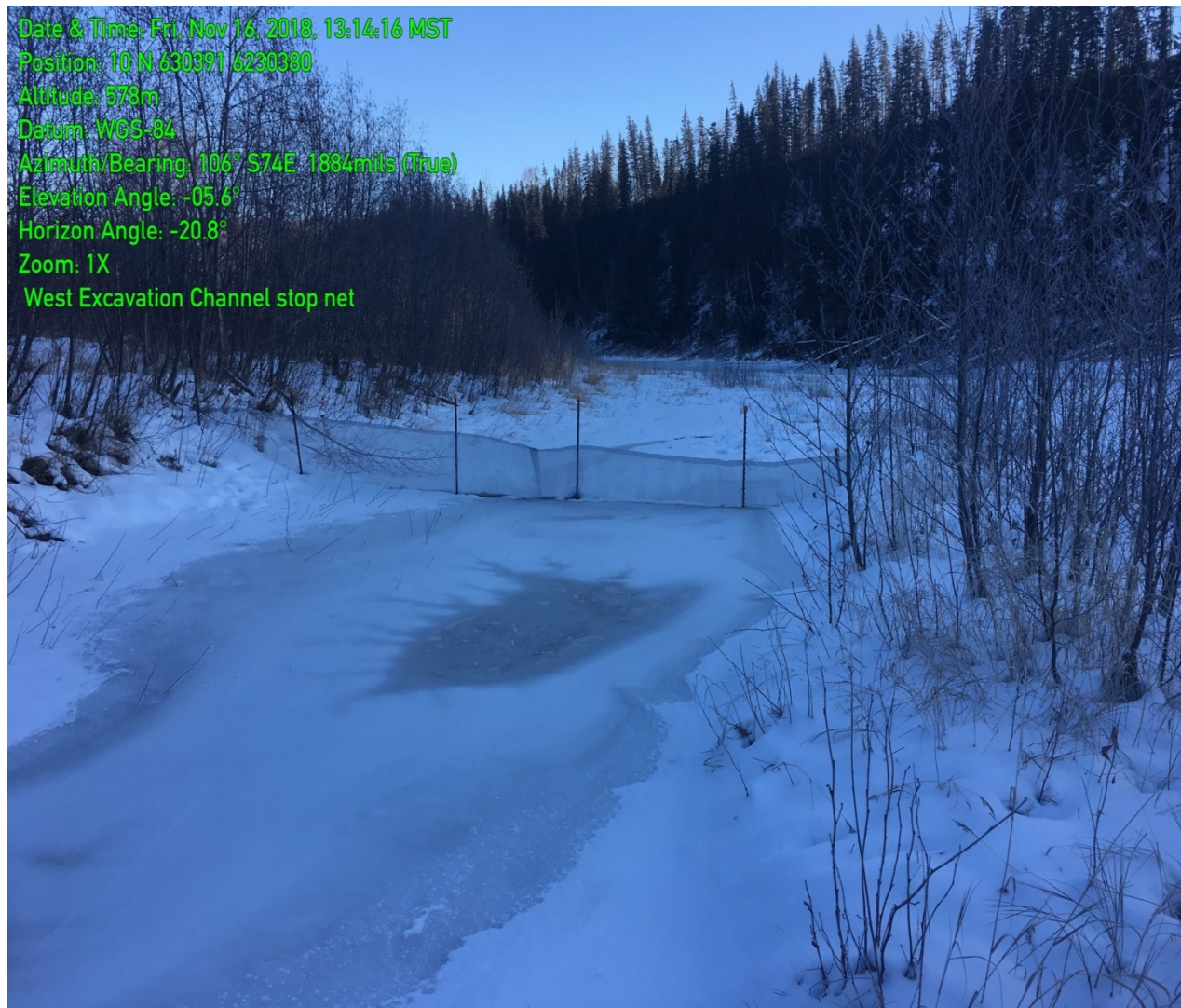
Figure 2. Fish were excluded using stop-nets during restoration of the back channel on the south bank island downstream of the dam (November 16, 2018).
