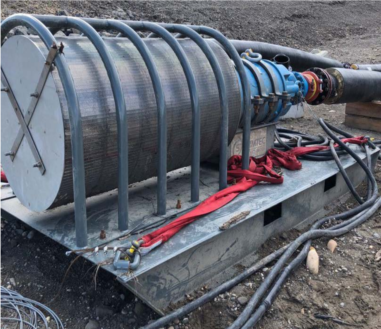
Figure 4. Water intakes were screened in accordance with Fisheries and Oceans Canada's Freshwater Intake End-of-Pipe Fish Screen Guidelines (July 2, 2018).
