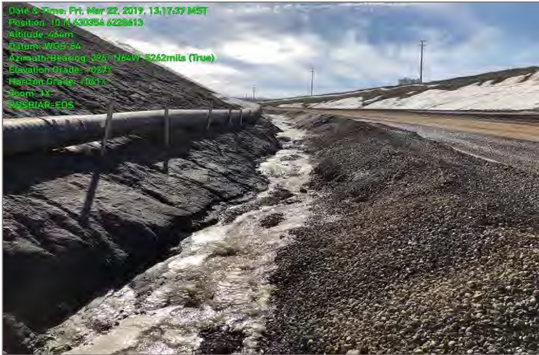
Photo 3: RBSBIAR-EDS east downstream ditch sample location looking south, dated March 22, 2019.
