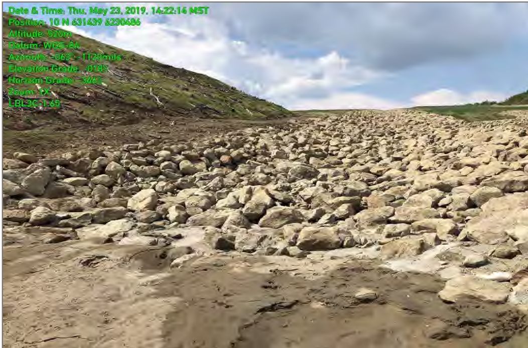
Photo 15: Spillway from RSEM L3, dated May 23, 2019.
