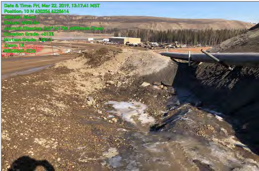
Photo 4: RBSBIAR-EDS east downstream ditch sample location looking north, dated March 22, 2019.
