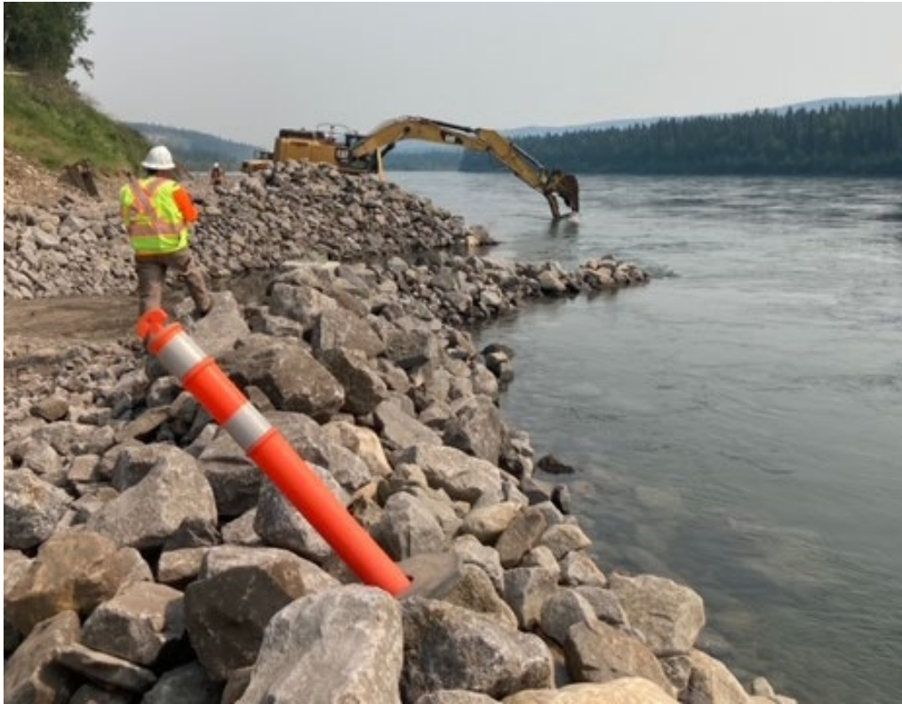
Figure 4. Fish habitat enhancement through boulder complex placement along the Hudson's Hope Shoreline Protection (August 15, 2021).
