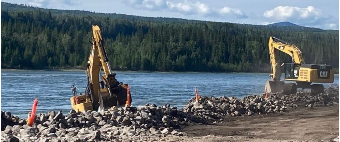
Figure 5. Riprap placement along Hudson's Hope Shoreline Protection (July 25, 2021). On site Qualified Environmental Professionals in place to ensure measures, including slow starts, controlled pace, and continuous of advancement, were being following to deter fish from active work areas.
