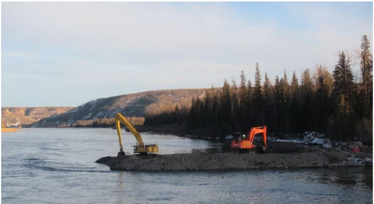
Figure 6. Temporary causeway used to support contouring of Peace River mainstem bar downstream of the dam site (January 17, 2021; from south bank looking east).
