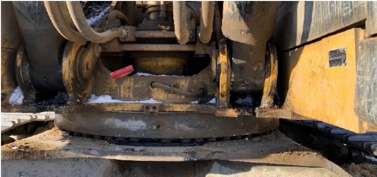
Figure 2. Within the dam site construction area all in-river machines are regularly checked for any signs of over greasing (February 3, 2021).
