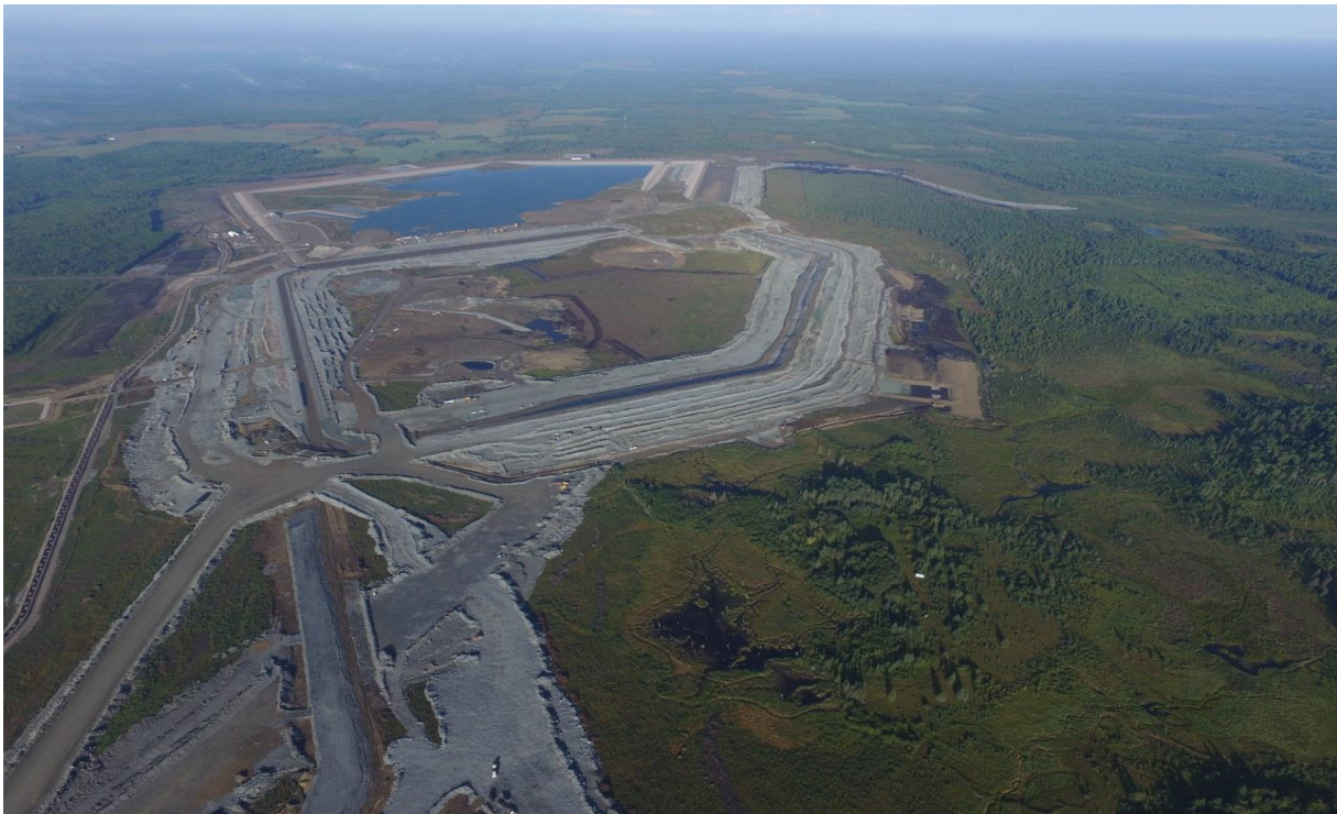
Figure 4: TMA facing west, September 2, 2017. Start up cell in foreground, water management pond in background
