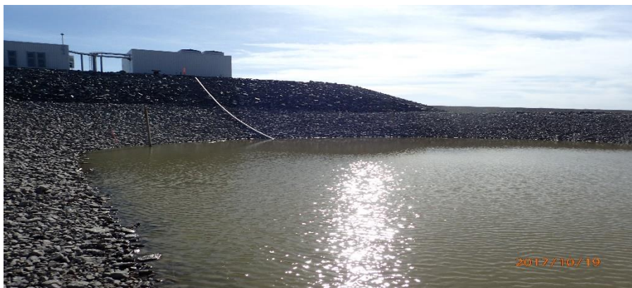
Figure 2: Water Management Pond Intake Structure, October 2017
