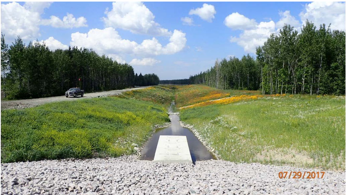
Figure 13: West Creek Diversion at the box culvert outlet, July 29, 2017
