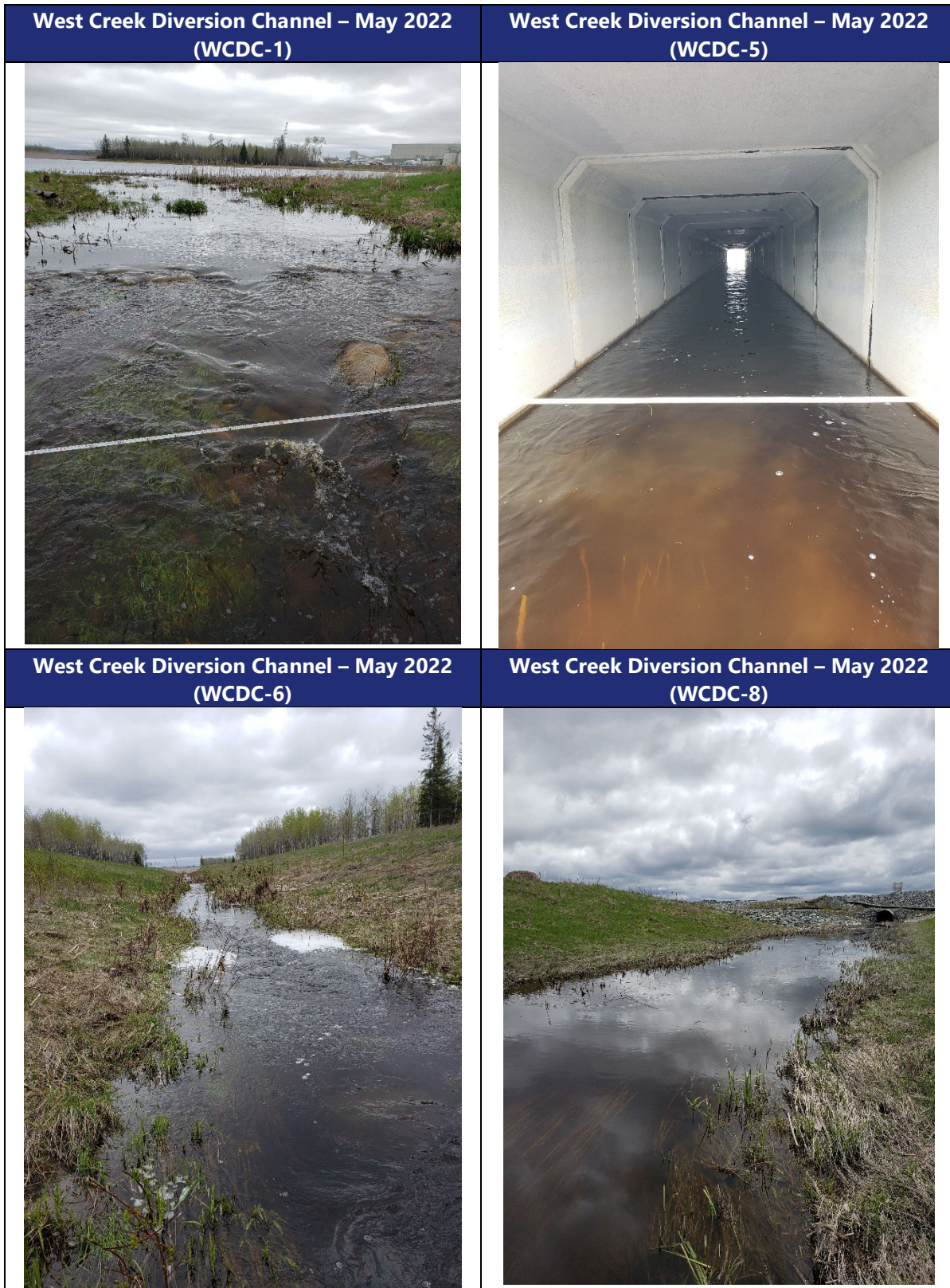
Figure B - 3: West Creek Diversion Channel (upstream of haul road), May 2022
