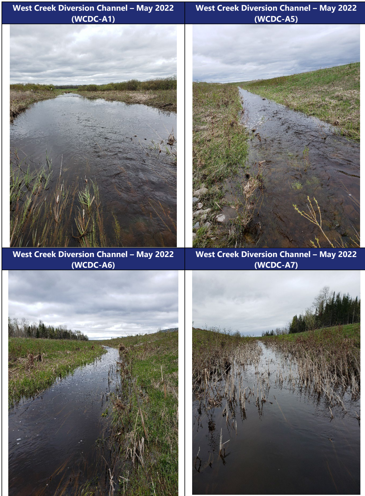
Figure B - 4: West Creek Diversion Channel (downstream of haul road), May 2022
