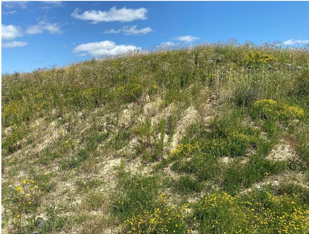
**Figure 6: West Slope Rill erosion.**
