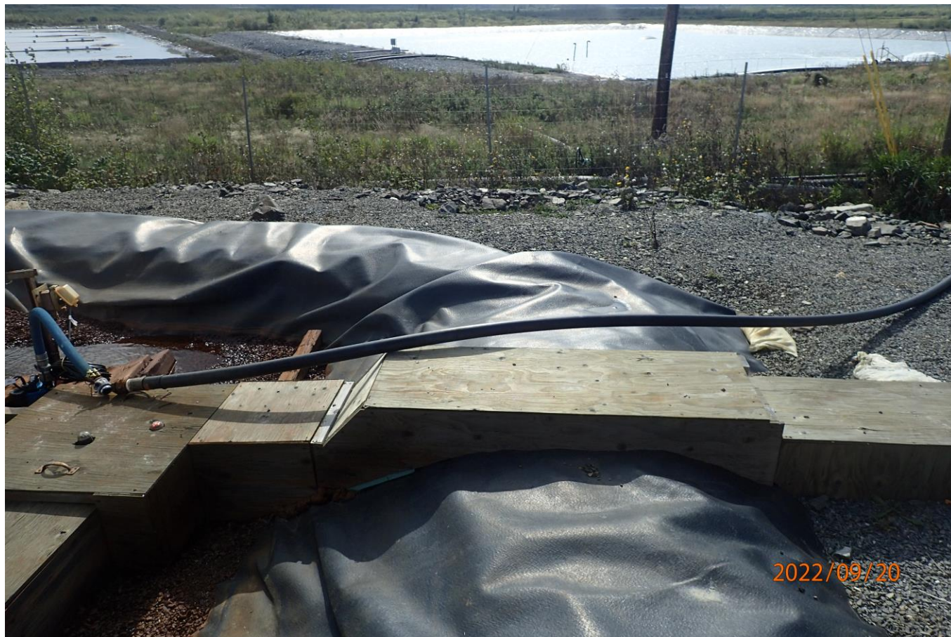
Photo 3: view of spill location from reagent tanks (BCR2 upper lefthand corner)
