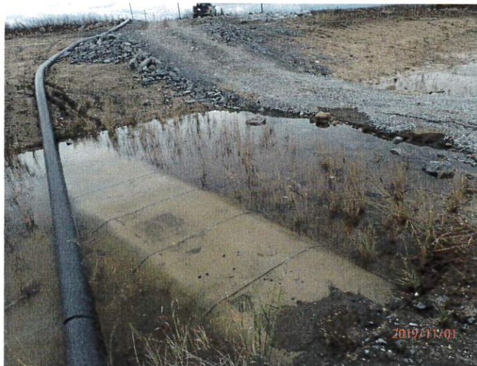
Figure 1 shows water flowing over sill in WDP Spillway and headed to remnant Loslo Creek.
