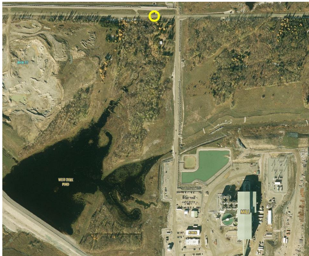
Figure 1. Plan view of plant site and West Creek Pond showing location of where the turbid water was spotted flowing under Roen Road.
