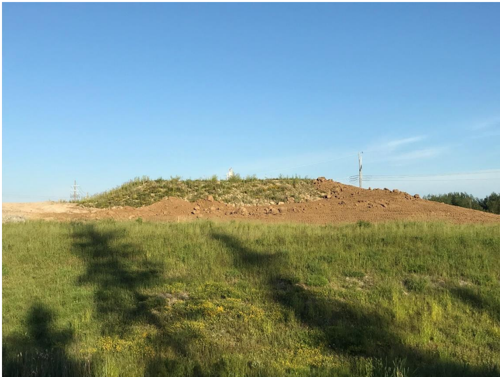
Photograph A.6: Material being added to east slope. July 15, 2019
