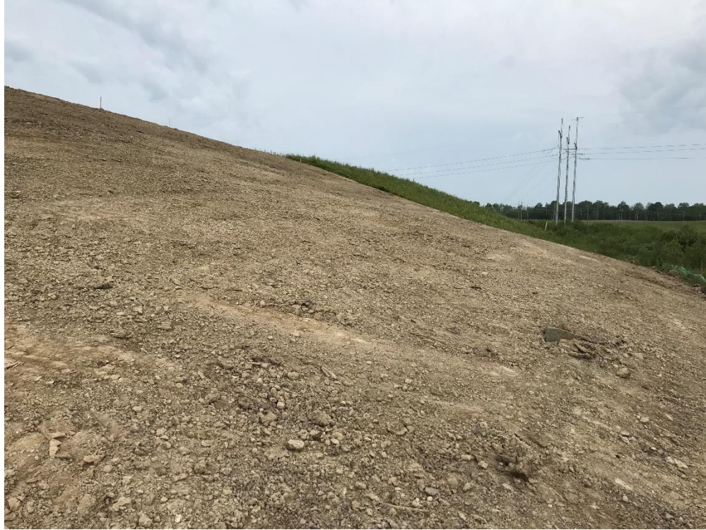
Figure 2.1: Completed modified north slope construction. July 17, 2019.
