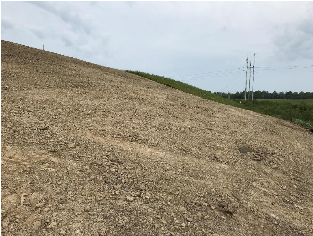
Photograph A.8: Completed north slope construction. July 17, 2019.
