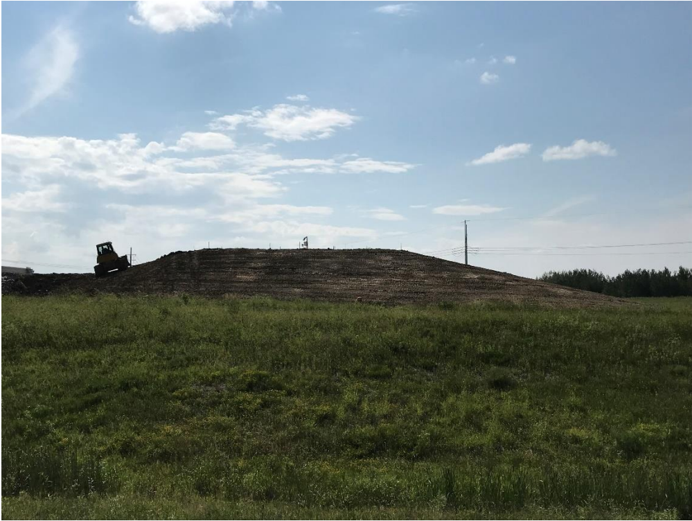
Photograph A.7: Completed east slope construction. July 16, 2019.
