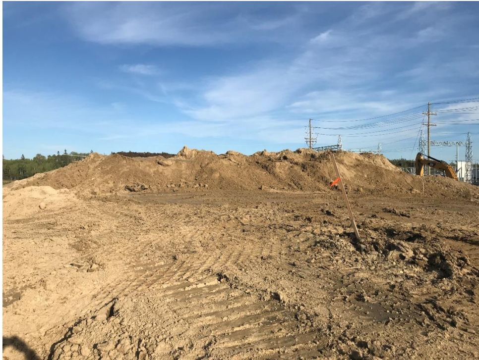
Figure 13: West slope plateau (destructive plot) area prior to grading material.
