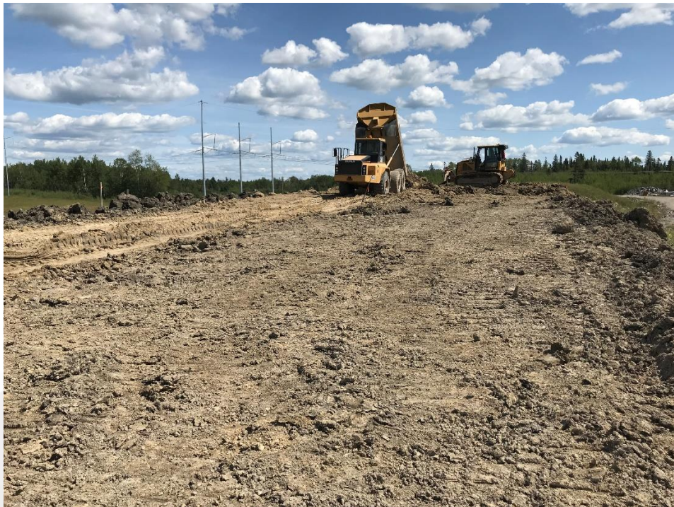
Figure 7: Hauling and blading cover system material on the plateau surface.
