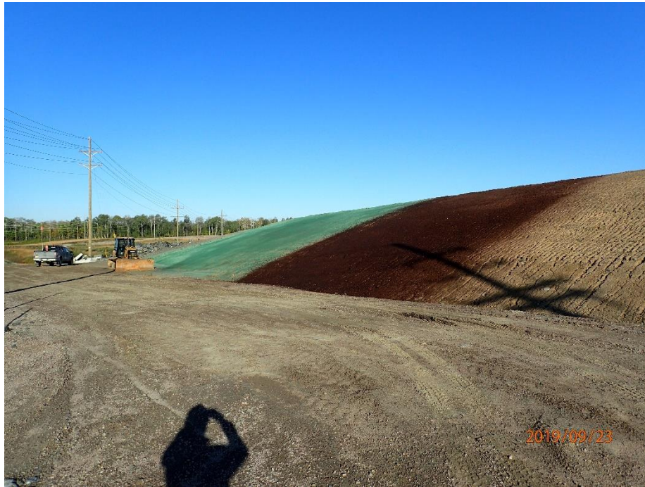
Figure 14: Landform slope following hydroseeding and application of ProGanics with unseeded control plot on right.
