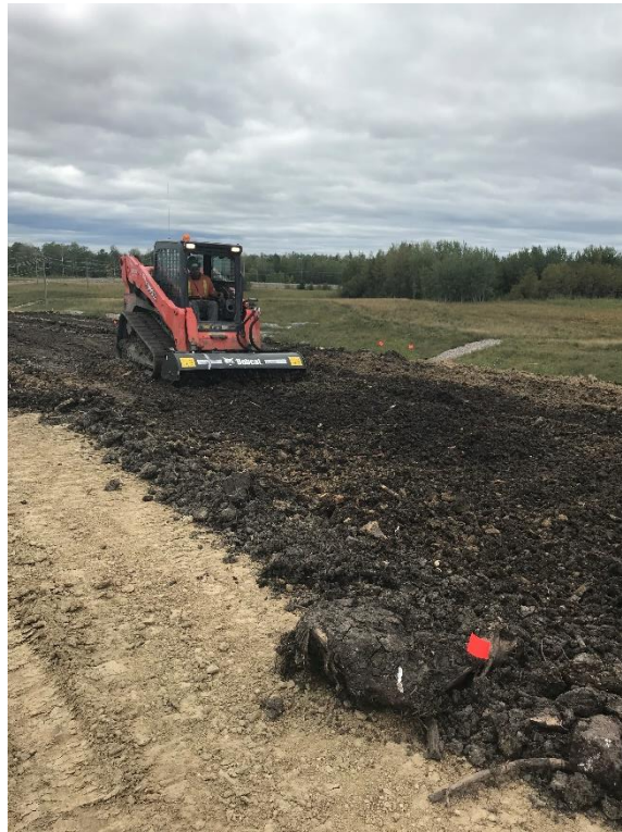
Figure 10: Topsoil incorporation into experimental plots using tiller attachment.
