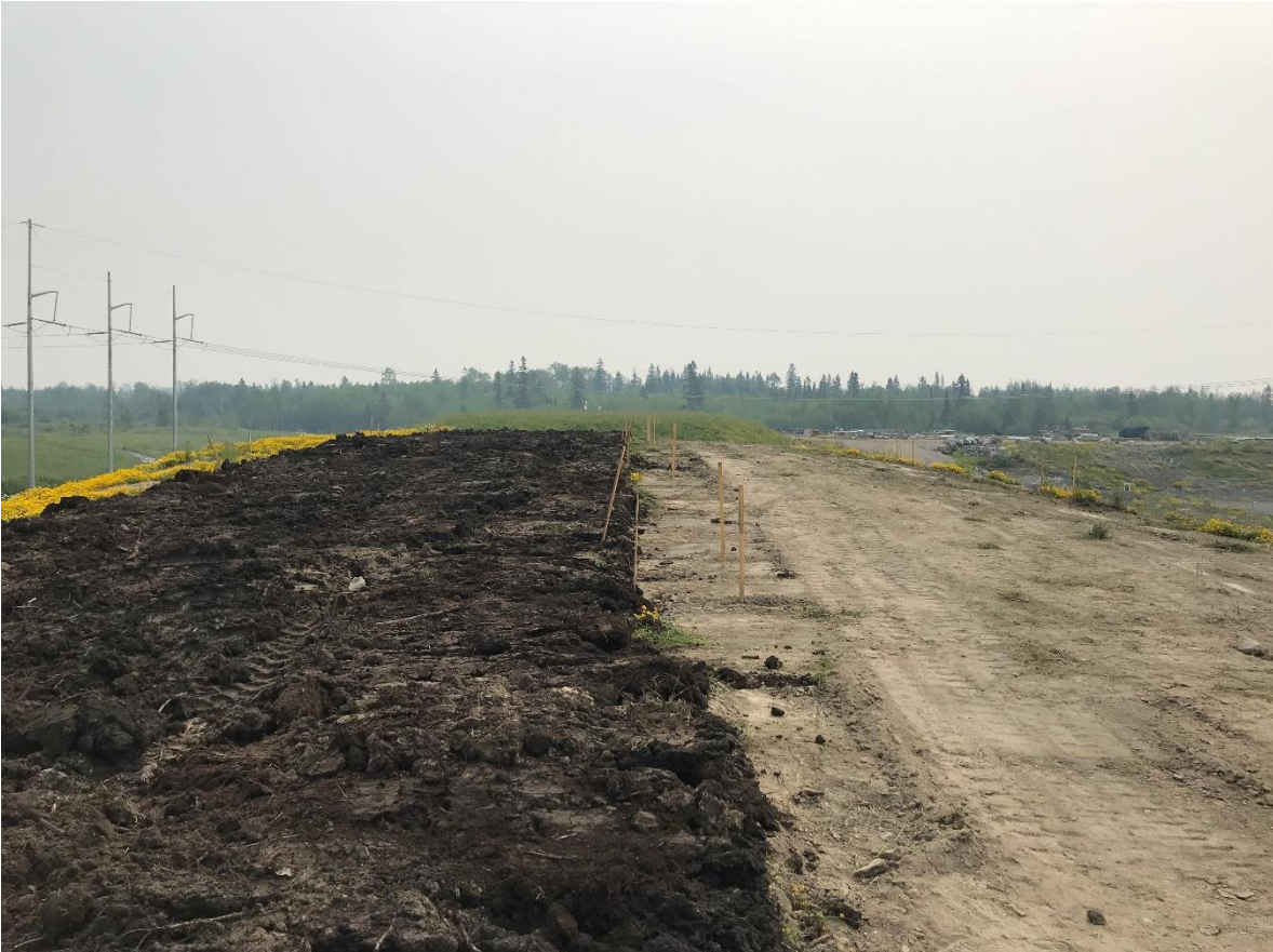
Figure 1: Initial plateau construction showing topsoil placement on the northern half of the plots (left side of figure).
