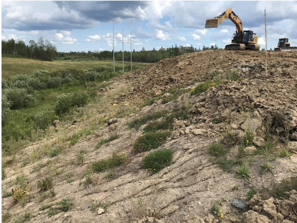
Figure 3: Construction of the north slope of the vegetation trial landform.
