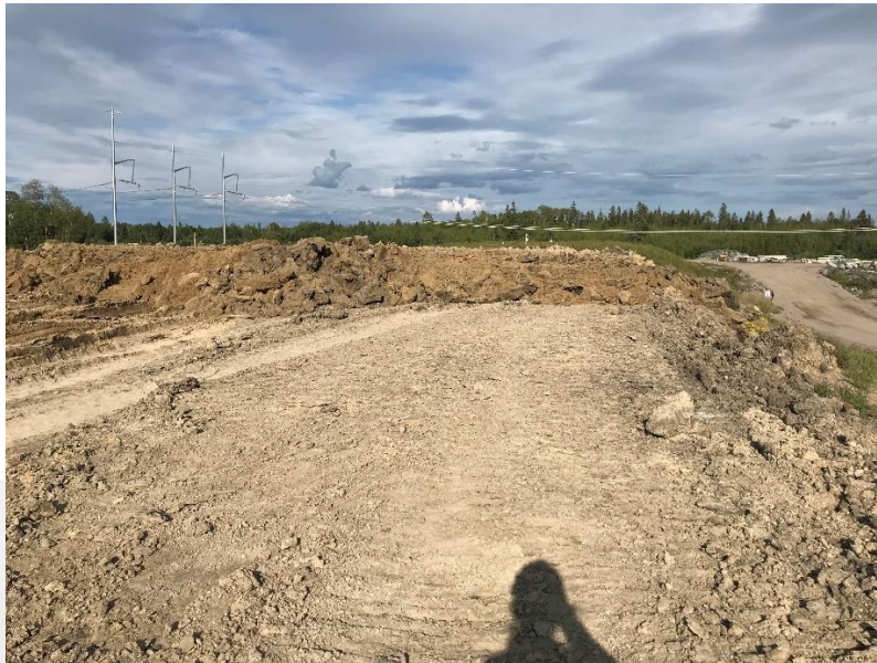
Figure 9: Placement of the overburden cover system on the plateau area.
