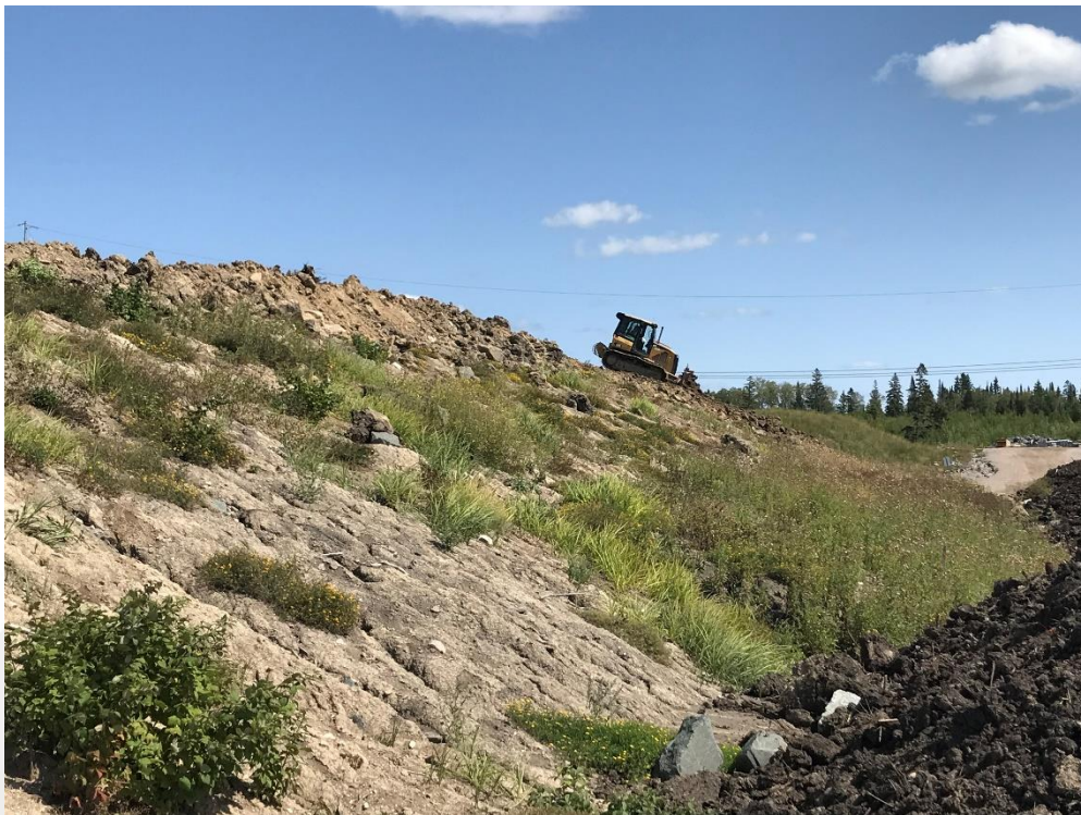
Figure 4: Construction of the south slope of the vegetation trial landform.
