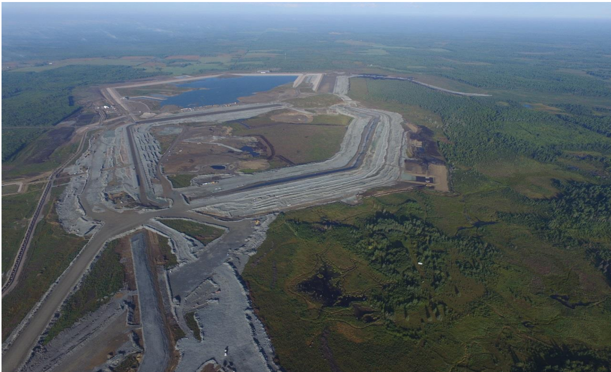
Figure 4: TMA facing west, September 2, 2017. Start up cell in foreground, water management pond in background
