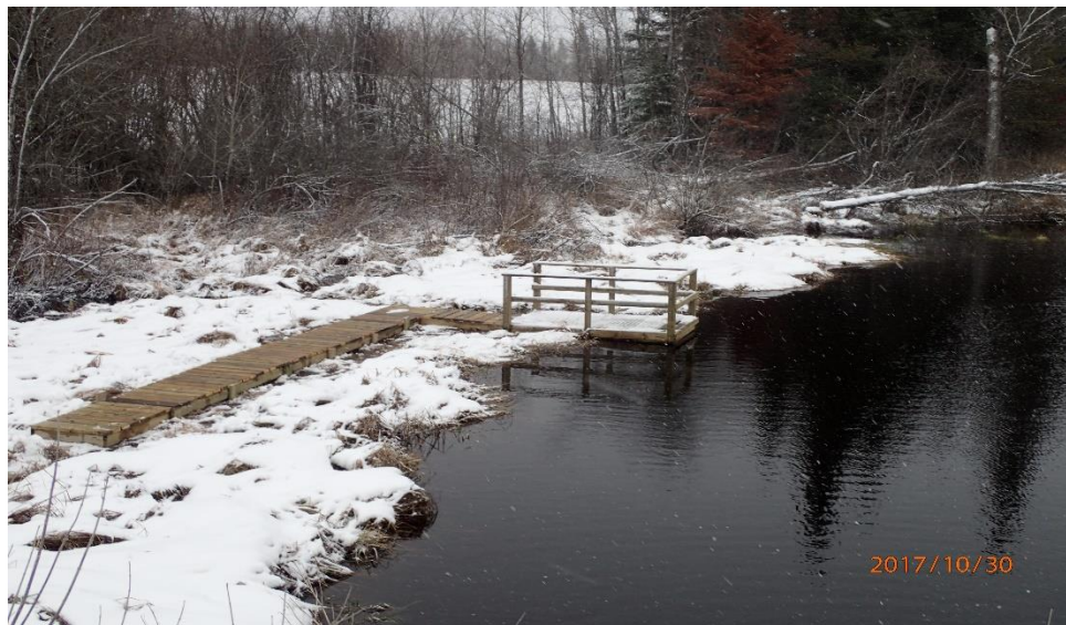
Figure 12: Water sampling platform installed on the Pinewood River
