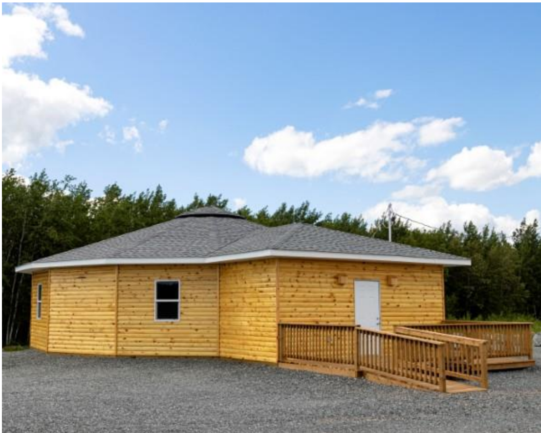
Figure 27. Newly built Round House on site
