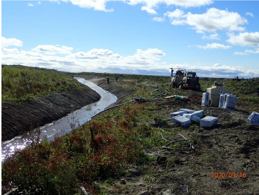
Figure 17. Hydroseeding the banks of Loslo Creek Diversion Ditch, September 2020.
