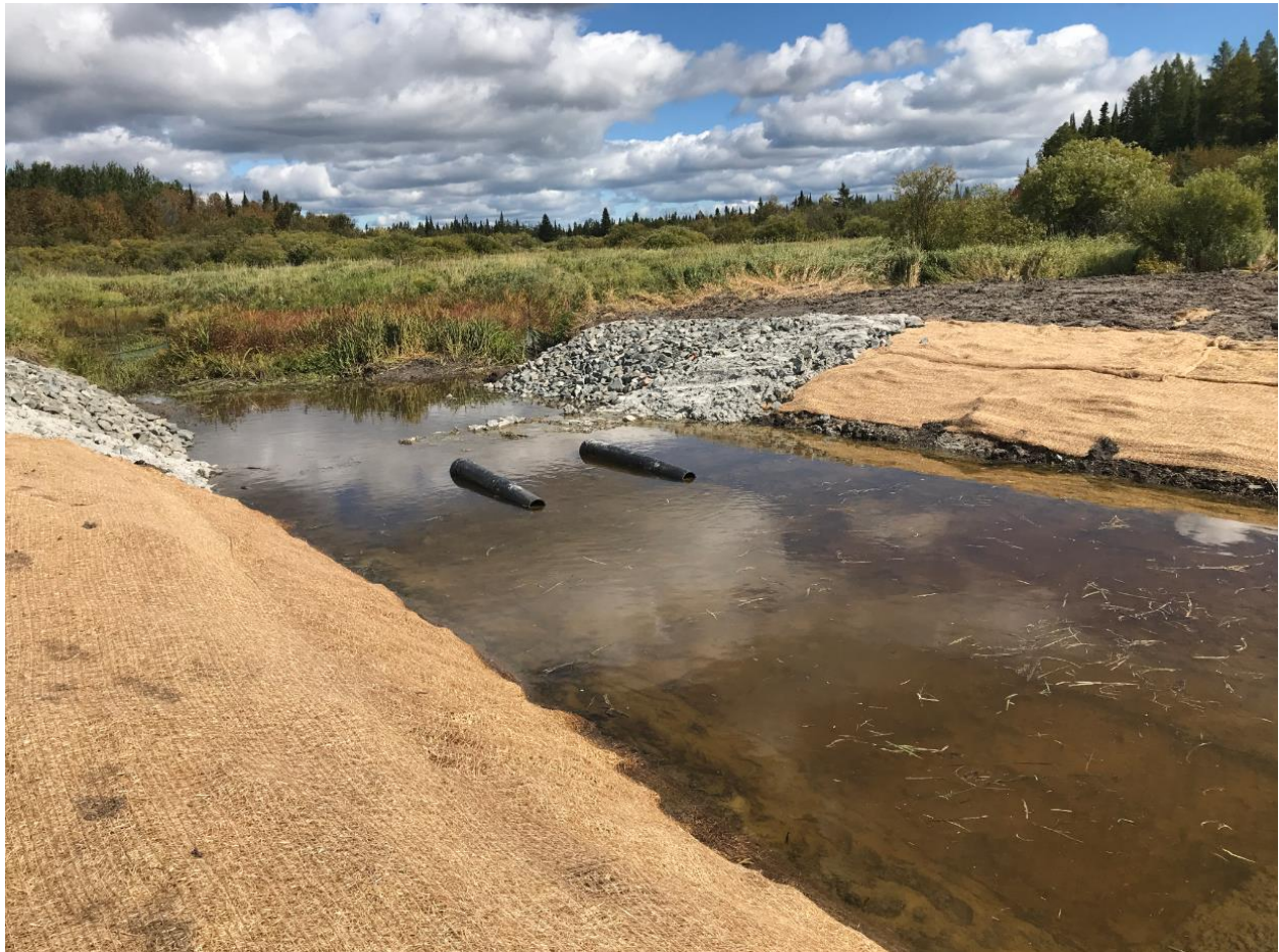
Figure 26. Diffuser construction complete at the Loslo Creek and Pinewood River confluence
