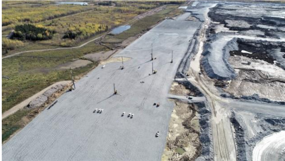
Figure 8. Wick drains installation program at the EMRS, 2020
