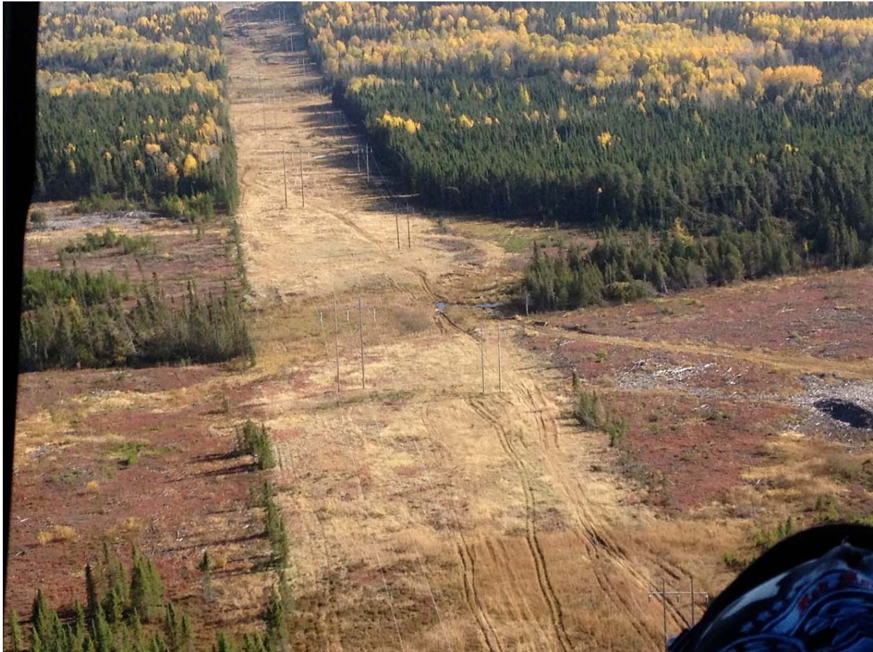
Figure 3.12-2: Power Line Infrastructure
