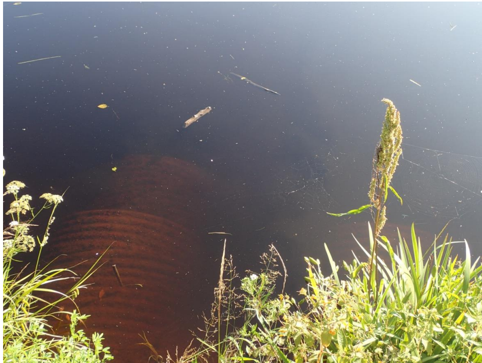
Figure 7. Upstream end of culverts underneath the railway that convey water from Blackwater Creek into Keplyn's Bay. August 3, 2016.
