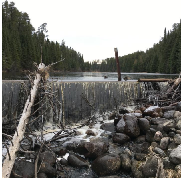
Figure 28. Dam at the downstream end of the Tree Nursery ponds on Thunder Lake Tributary 3. April 24, 2017.
