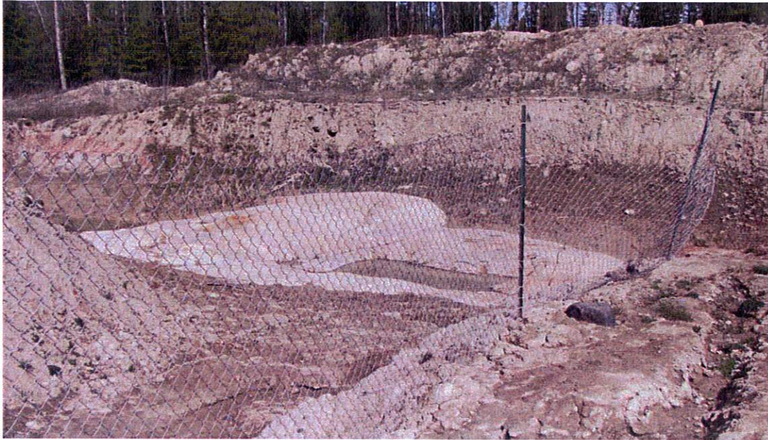
Image 17. View north above Beaver Dam of exploratory location and clay covered bedrock.
