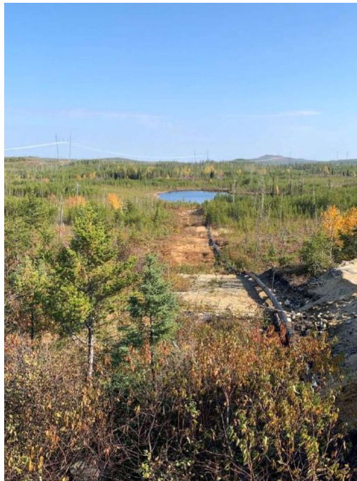
Figure 2-2. Discharge Line Leading to the Small Lake (petit lac)
