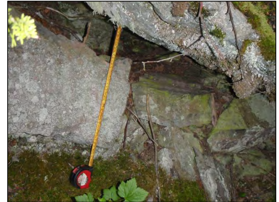
Photo 23: Fractured rocks observed at 68med
