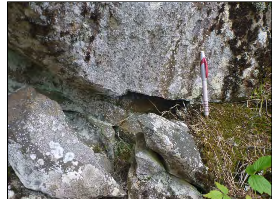
Photo 12: Crevice observed at 115lo
