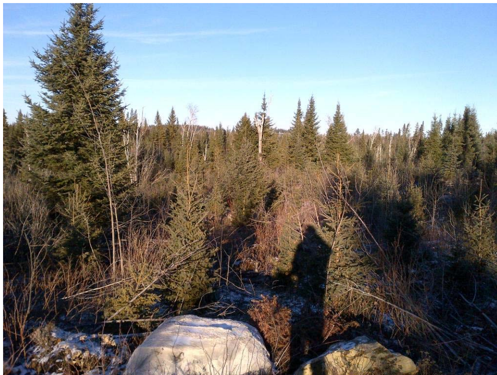
Photograph 36: TMF South Dam Perimeter Looking East
