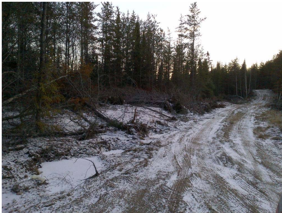
Photograph 31: Process Plant Location
