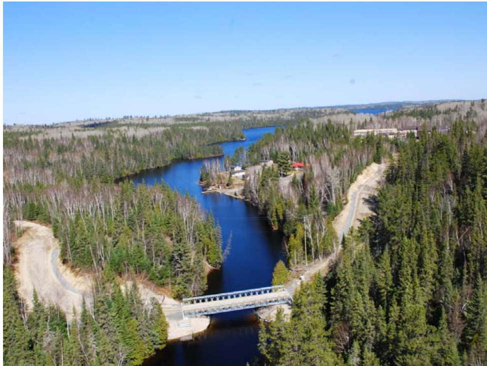
Photograph 42: Bridge Crossing Mesomikenda Lake and Exploration Lodge and Camp
