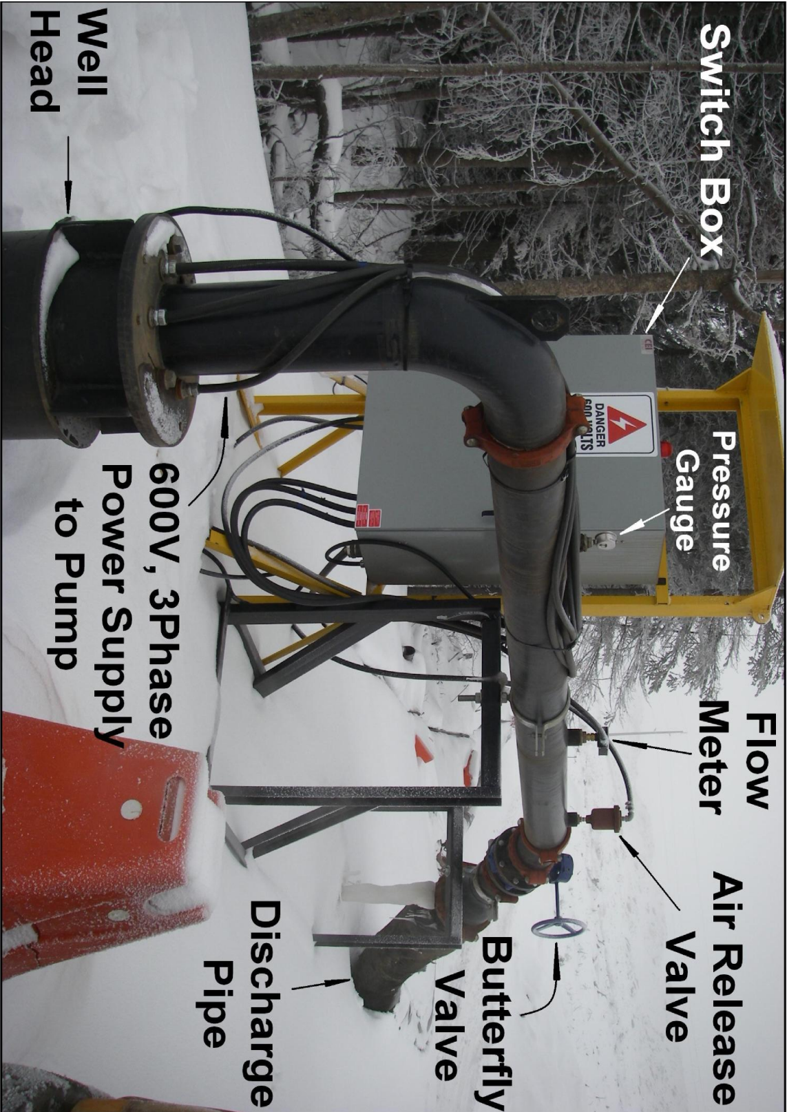
Figure 2.15 Typical Layout for a Groundwater Extraction Site
