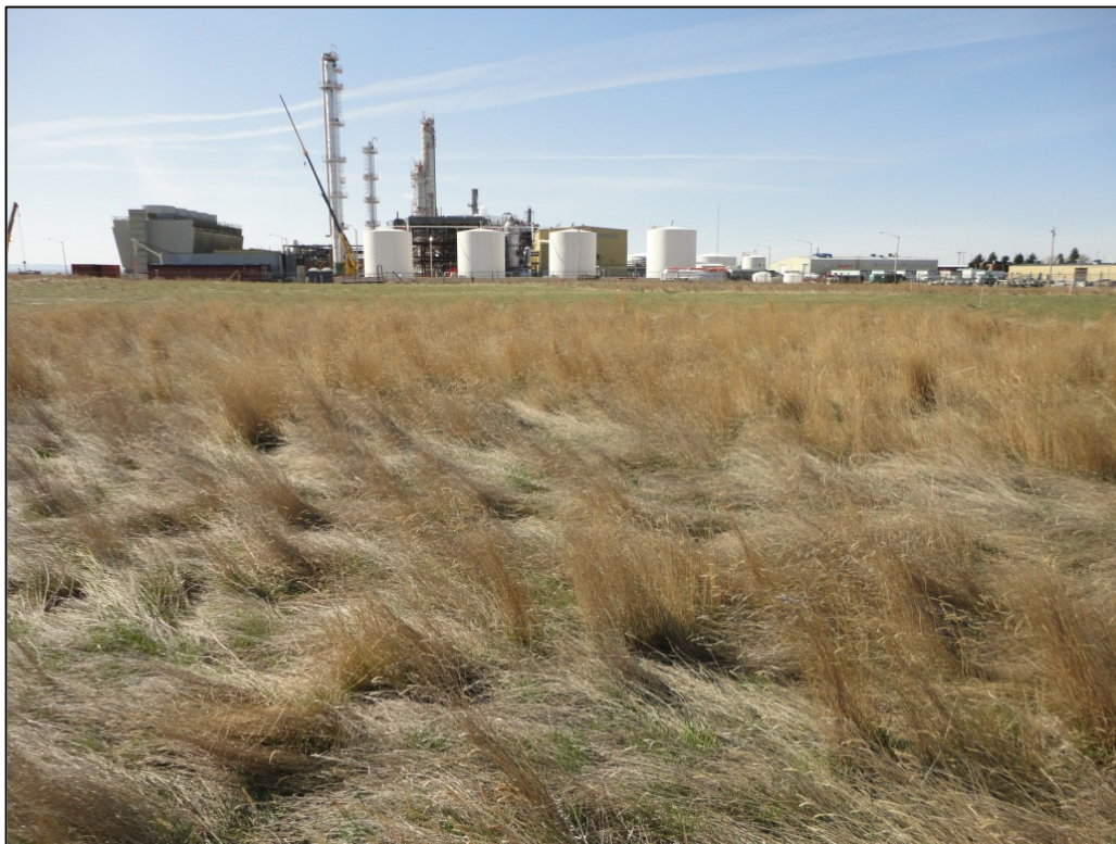
Figure 8 - Central Location Viewing South (existing Methanex infrastructure in background)
