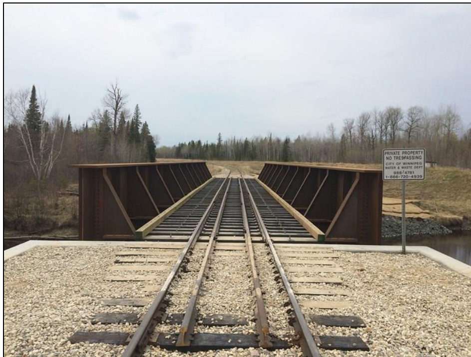
Figure #6 – Typical Steel Open Deck Through Plate Girder Bridge
