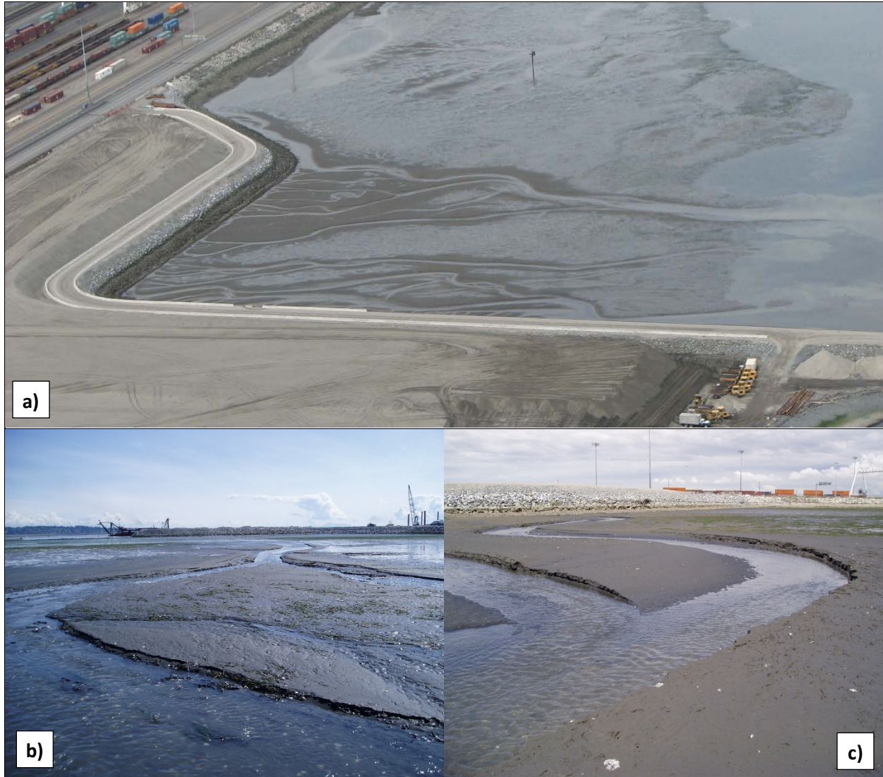
Figure A-6 a) Aerial view of DP3 tidal channels (photo taken 12 March 2008 during project construction); b) and c) show various segments of the channels from the ground (photos taken 18 April and 14 June 2007, respectively).
