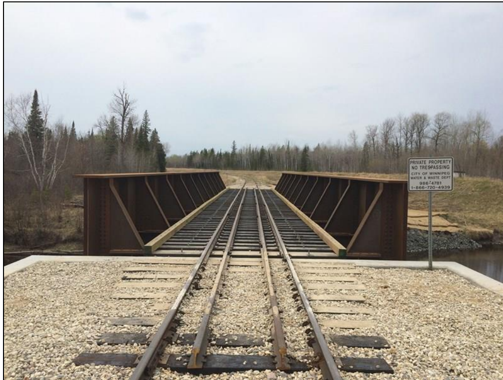
Figure #1 – Typical Steel Open Deck Through Plate Girder Bridge
