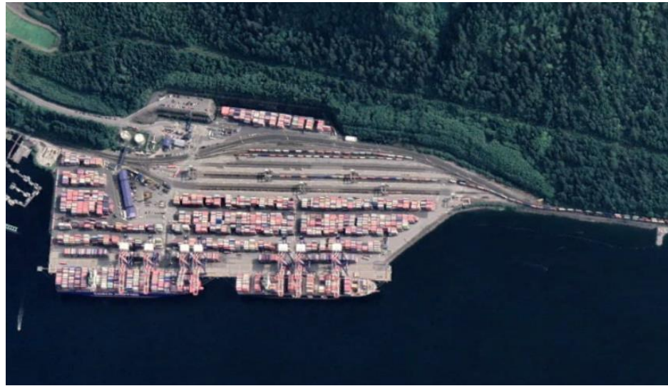
Google Earth view of Fairview Terminal (September, 2020)
