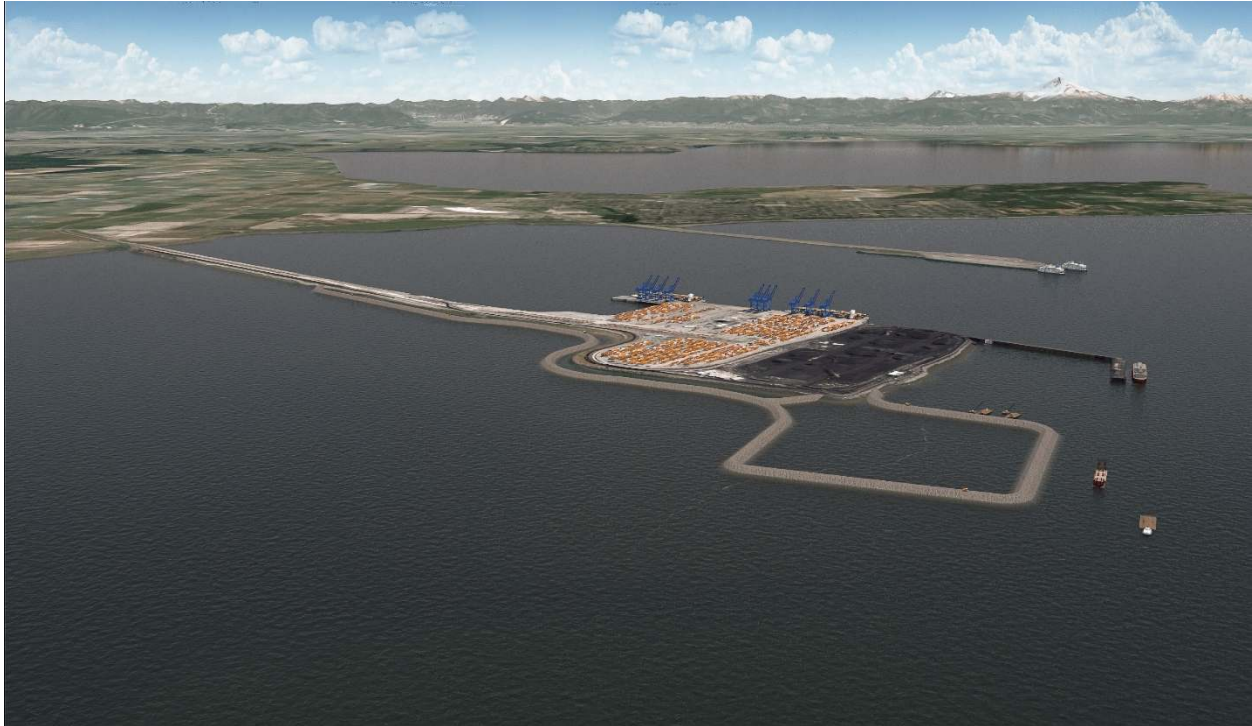
Figure 1. East containment dyke constructed: monitoring implemented at this juncture.*
