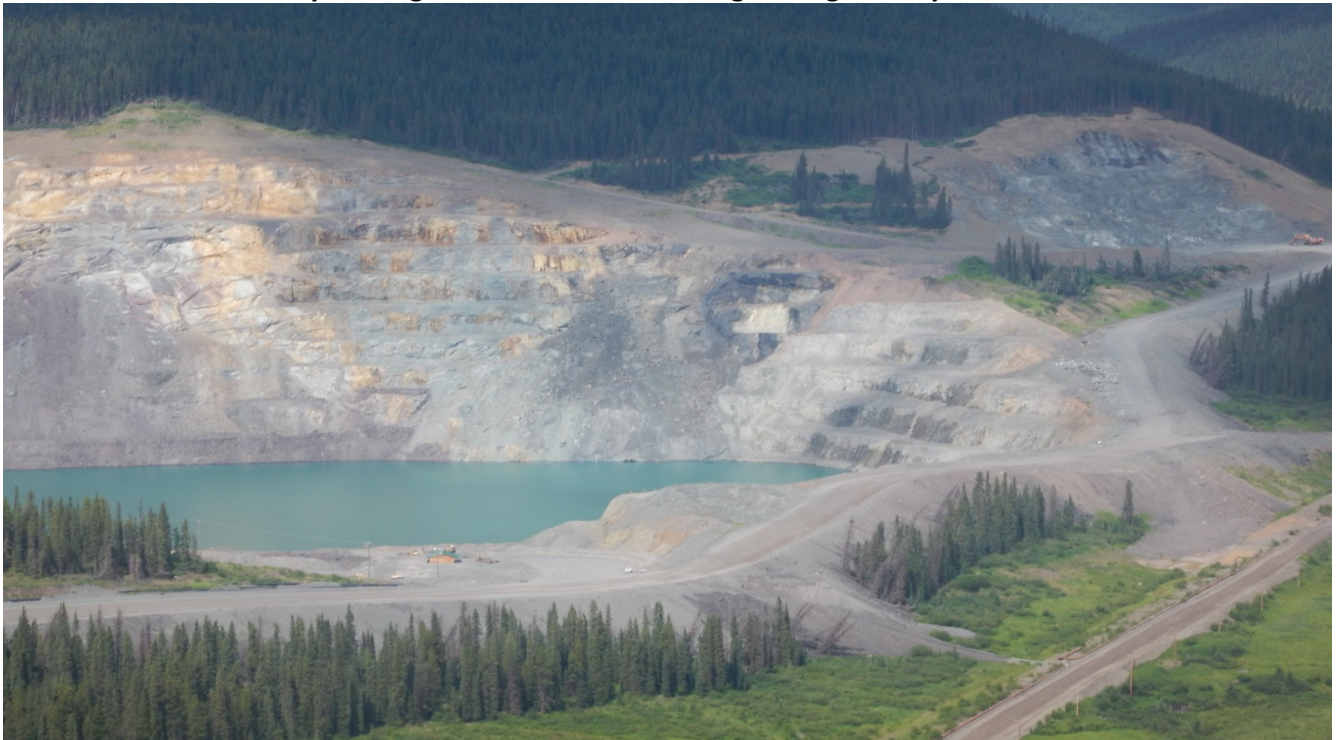
Plate 3.6-1 East Pit Quarry Drainage area into the KUG tailings storage facility
