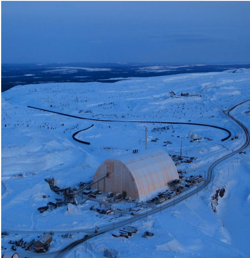
Dôme – Dome Completion
