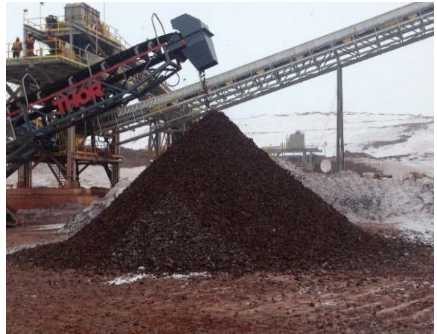
Dry processing facilities Commissioned
