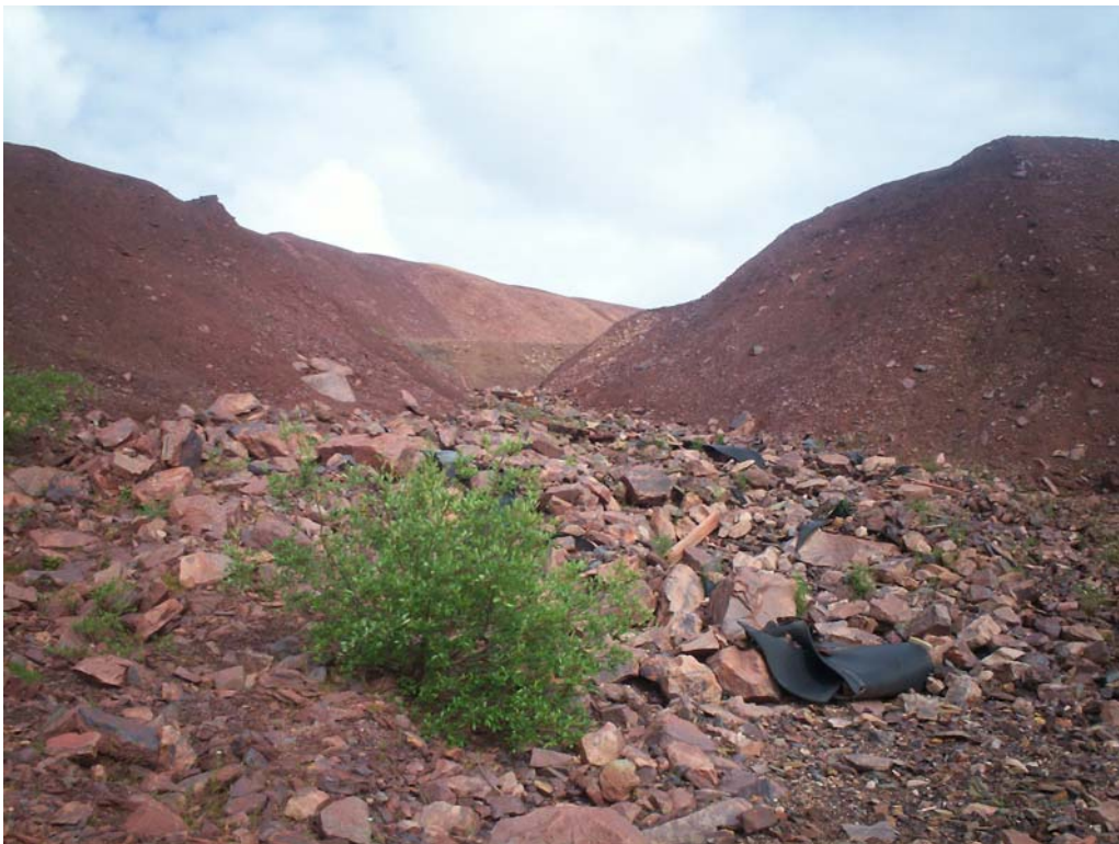
Photo B-48. Timmins 1 Ditch, upstream view (a lot of debris such as wood and rubber conveyor belts in ditch)
