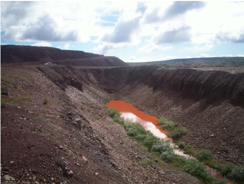
Photo B-46. Timmins 1 Ditch, upstream view from road which runs to Timmins 1 (could not find culvert inflow on other side of road)
