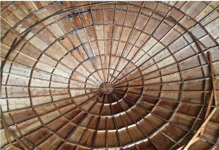
Photo 3: Sand Dome interior
