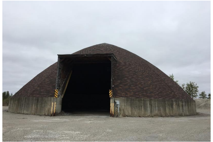
Photo 2: Sand Dome exterior
