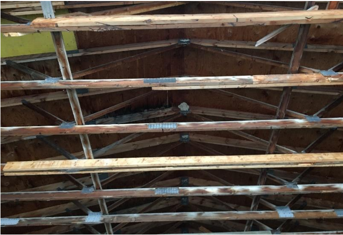
Photo 7: Garage Interior. Barn Swallow Nest Visible.
