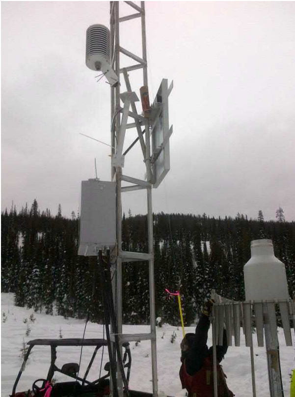
Photo 1. Crown Mountain Climate Station Installation (November 29, 2013)
