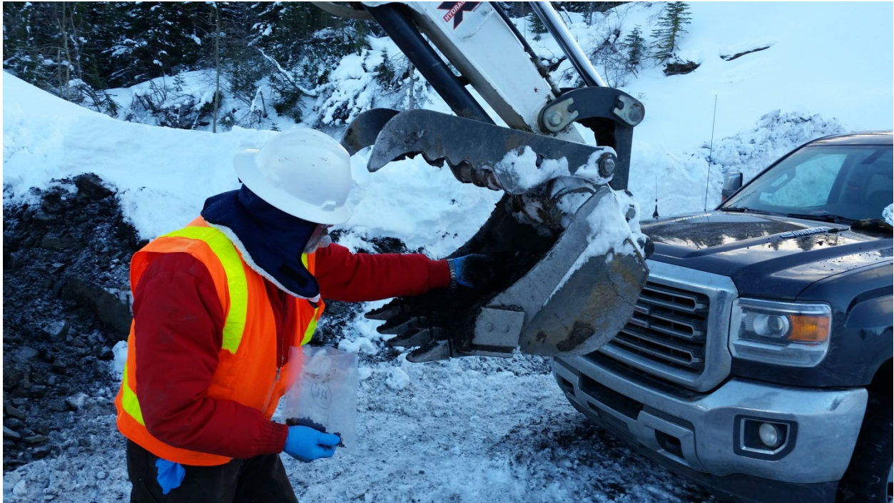
Photograph 6. Samples being hand-selected for fines from the mini-excavator bucket by Enviromin. Photograph looking southeast. November 30, 2017.
