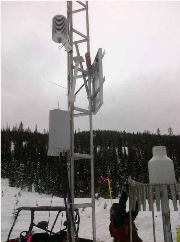
Photo 1: Crown Mountain Climate Station Installation (November 29, 2013)
