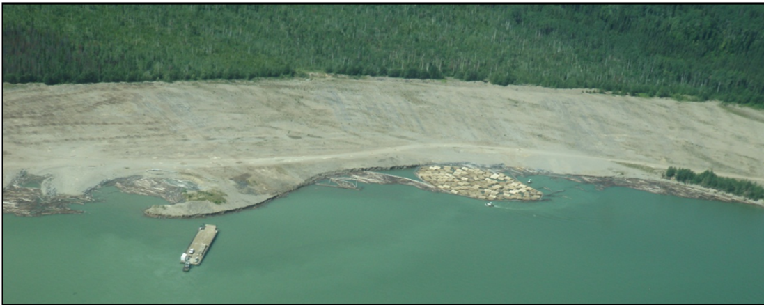
Photograph 5 – the existing barge landing and access road at Ospika.
