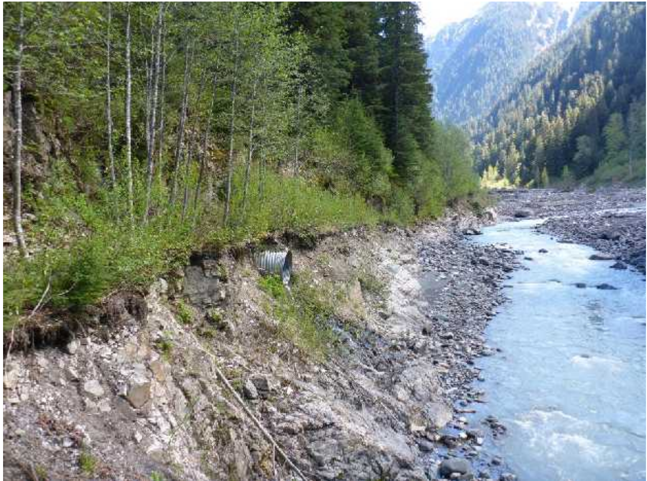
Figure 2: Upstream view at of road encroachment area in a confined section of Bitter Creek. The culvert inflow on river right, conveys a tributary watercourse ( i.e. road crossing). Date taken: 16-May-2017.
