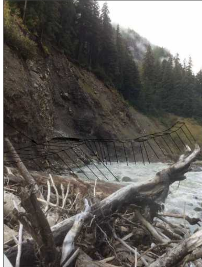
Figure 5: View of upstream section of road encroachment area. Source: Onsite Engineering, Drawing # 1464-2-RIVERFILL- 002
