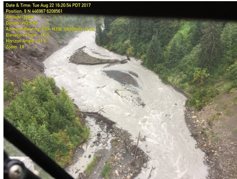
Photo 2: Bitter Creek Road Interference Area (station 4+550 m to 4+840 m), August 22, 2017
