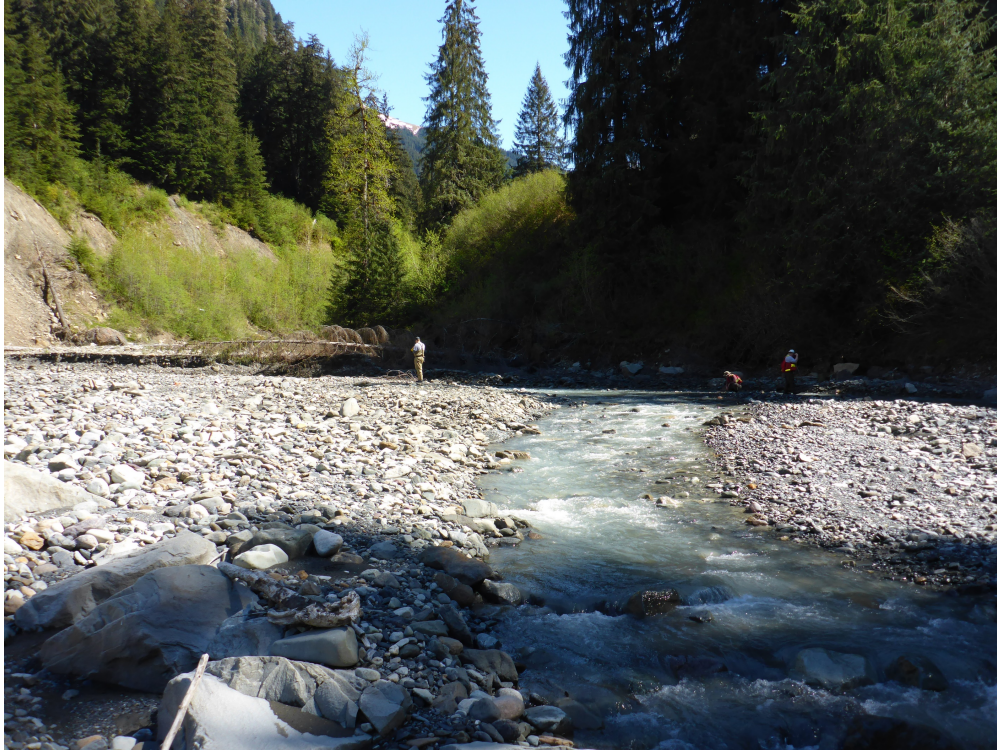
Photo 5: Bitter Creek Road Interference Area (station 4+550 m to 4+840 m), showing side channel on river right (looking upstream) May 16, 2017
