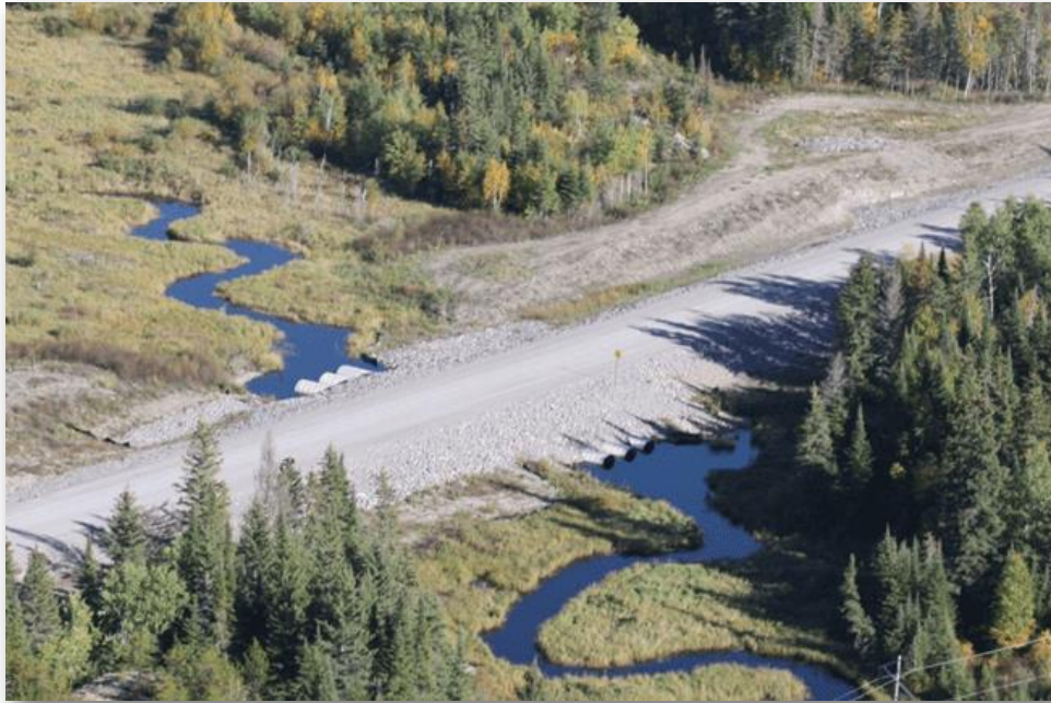
Photograph 3-3: Typical Multi-Culvert Stream Crossing
