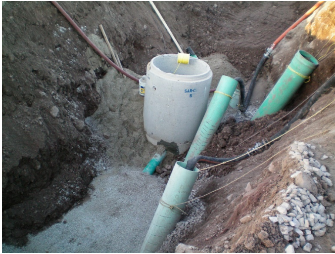
Photo 1: Example of pumping from filtered sumps within excavation areas
