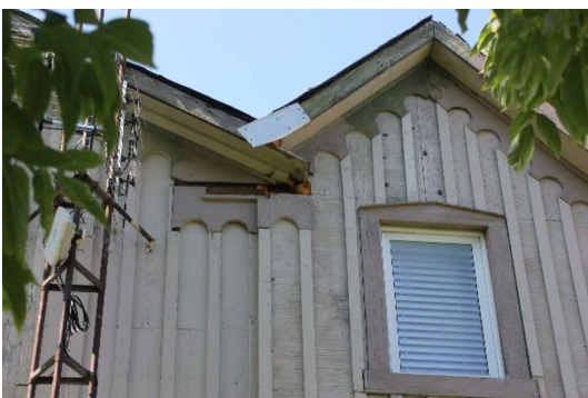
Plate 10: Board and batten siding and decorative wooden trim and window surrounds, southeast façade, looking west
