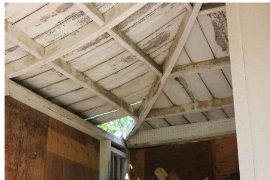
Plate 5: Rafters under covered porch on southwest façade, looking west
