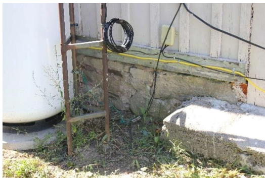
Plate 9: Stone foundation, southeast façade, looking west
