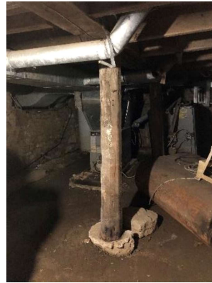
Plate 13: Timber support beams on concrete footing
