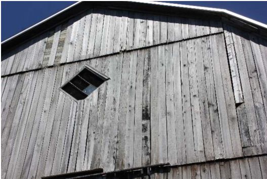
Plate 18: Southwest façade, looking north
