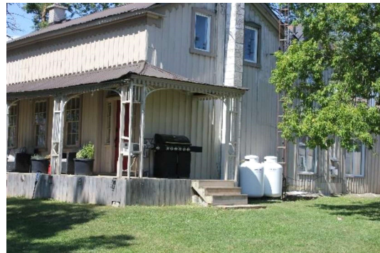
Plate 7: Southeast façade, looking northwest
