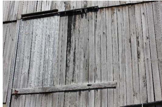
Plate 19: Sliding door and vertical timber cladding, southwest façade, looking north
