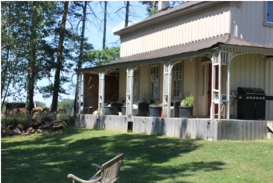
Plate 2: Southwest façade, looking northwest
