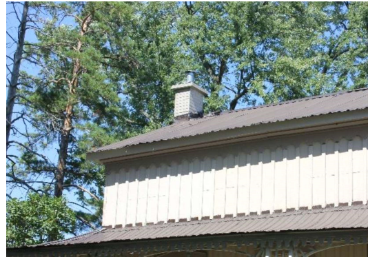
Plate 3: Buff brick chimney, looking northwest
