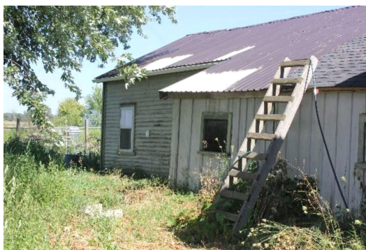
Plate 11: Northwest facade, looking northeast
