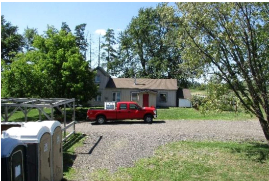
Plate 6: Southeast façade, looking northwest
