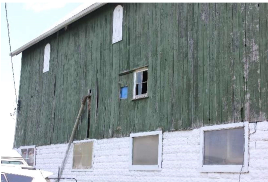
Plate 20: Northwest façade, looking northeast
