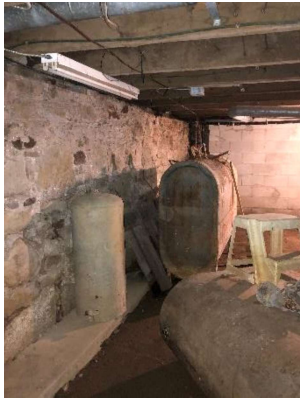
Plate 12: Stone foundation and concrete block walls in basement
