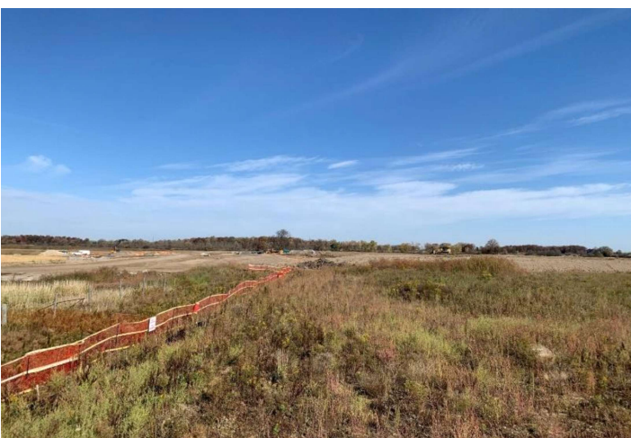
Photo 9: 5381 Tremaine Road, Milton - Construction Soil Sampling Location T-SS-02 – Located in Construction Area beside Orange Fencing
