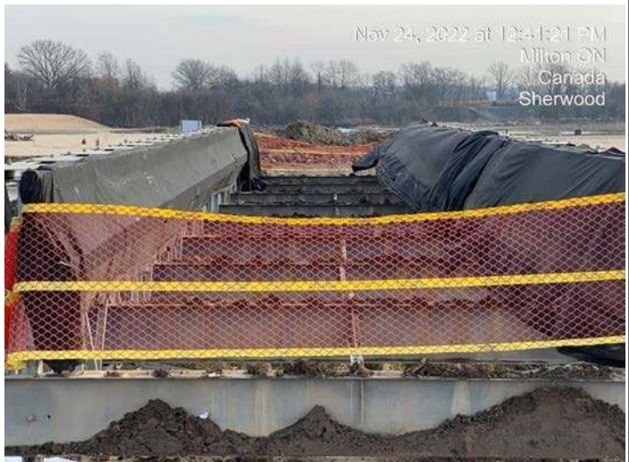
Indian Creek - Dismantle and remove bridge decking
