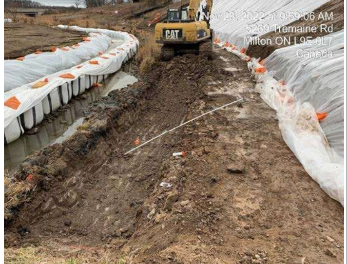
Pond 2 Area Enhancement - Excavation of material for Riffle installation
