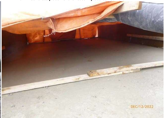
Trib. A - Finished surface cast in place box culvert section 2A
