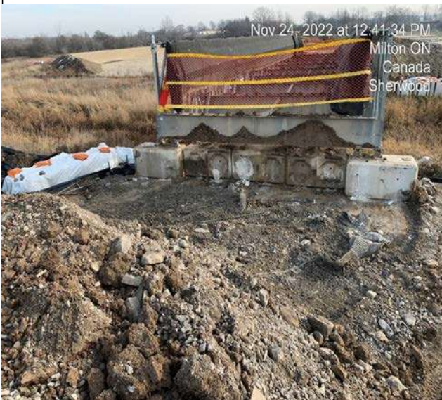
Indian Creek - Dismantle and remove north abutment materials from bridge
