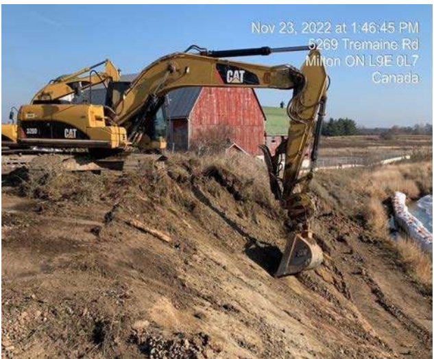
Pond 2 Area - Excavation of material for slope grading
