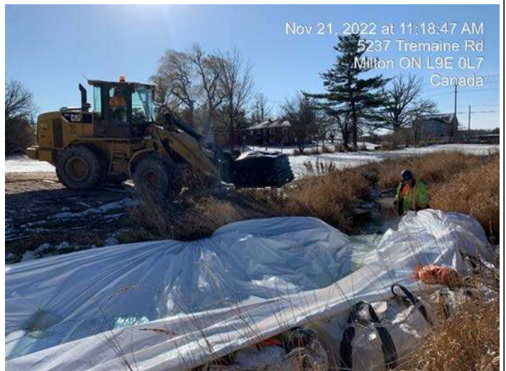
Pond 2 Area - Installation of poly tarps and sand bags for coffer dam
