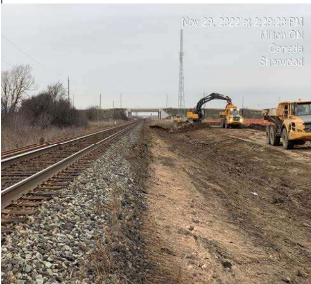
North Crossing Area - Continue striping and grading along ROW
