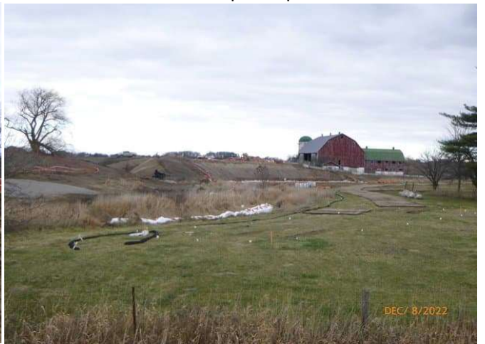
Indian Creek - Installed cofferdam for next enhancement section
