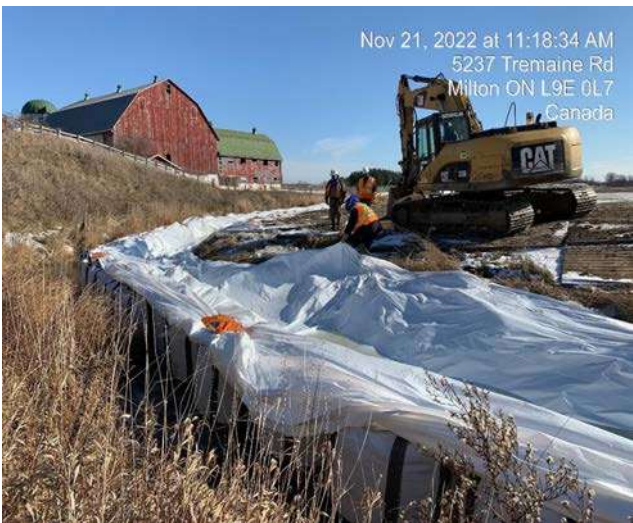
Pond 2 Area - Installation of poly tarps and sand bags for coffer dam
