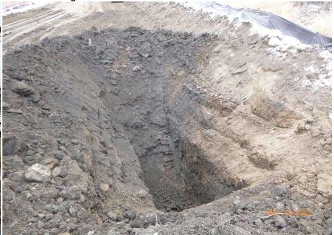
Track Realignment - Identified organic material South of Trib. A
