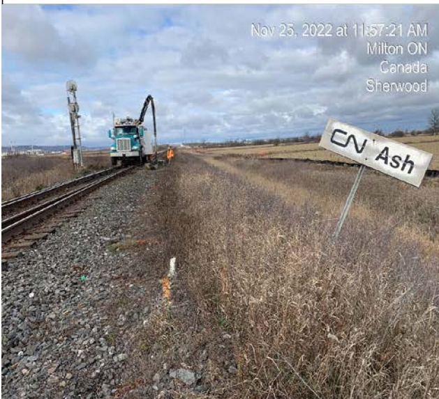
North Track Crossing - Hi-Rail vac truck locating signal cables along ROW
