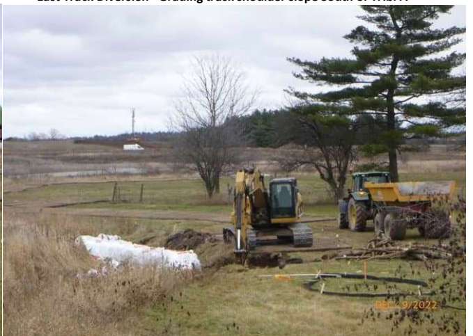
Indian Creek - Excavation for wooden toe debris enhancement section
