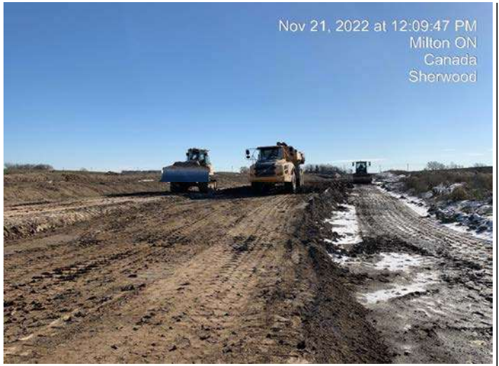
East Track Diversion - Excavation and grading for track diversion grading
