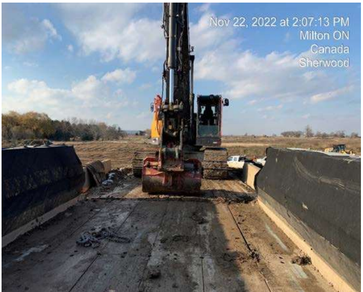
Indian Creek - Begin dismantle south approach sections at bridge
