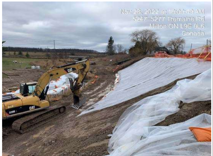
Pond 2 Area Enhancement - Poly tarped protected slope.
