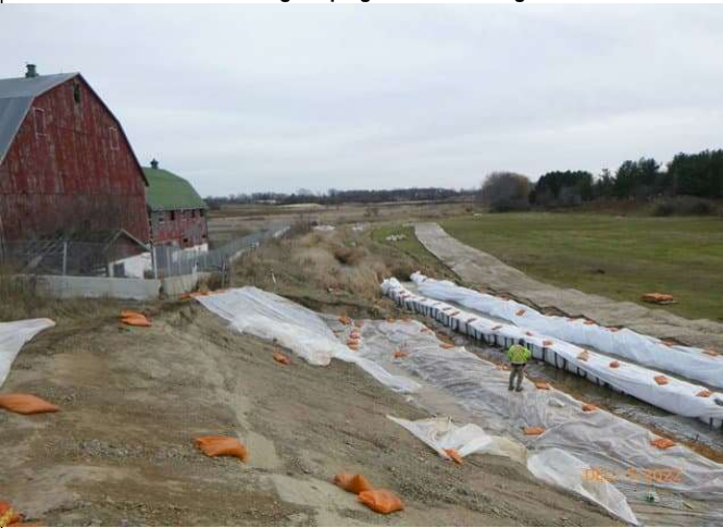
Indian Creek - Wooden Toe Protection construction along enhancement areas
