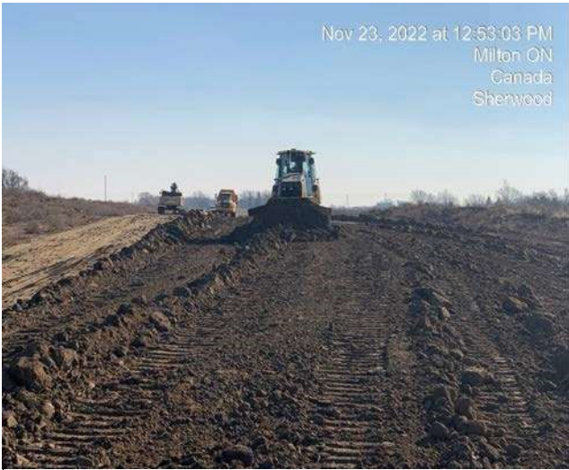
East Track Diversion - Grading of cut/fill material for track diversion
