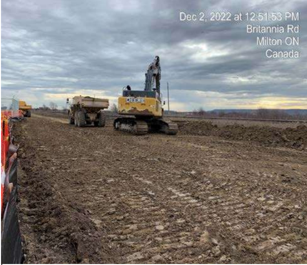
North Crossing Area - Continue striping and grading along ROW
