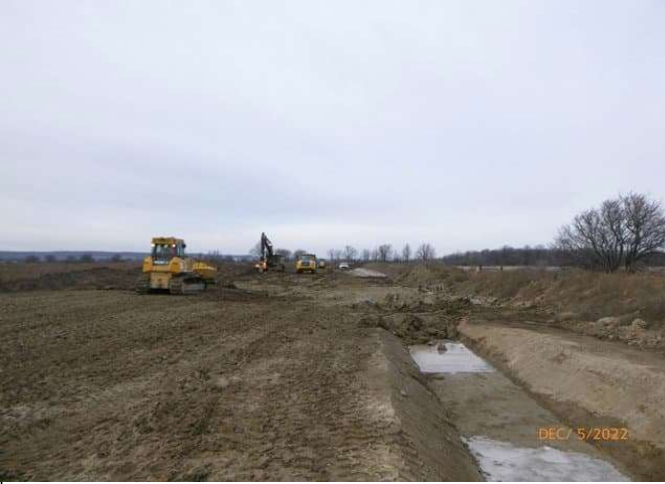
East Track Diversion - Grading/shaping ditches heading North to Trib. A
