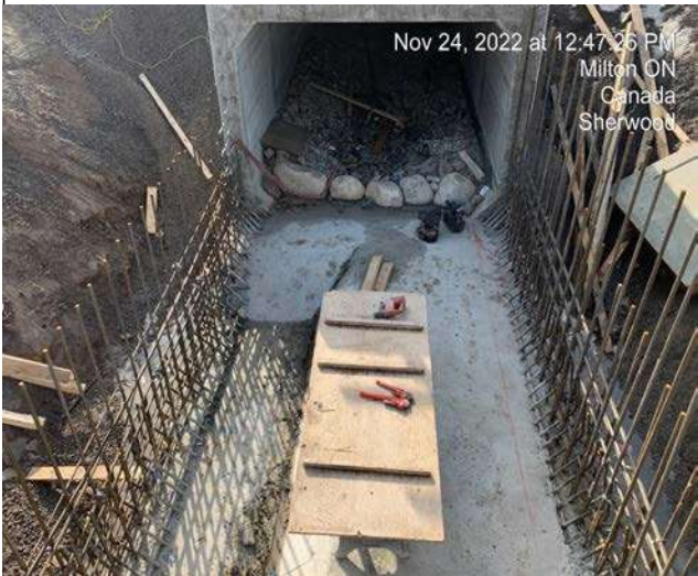
Trib A Box Culvert - Continue works on Cast in Place section
