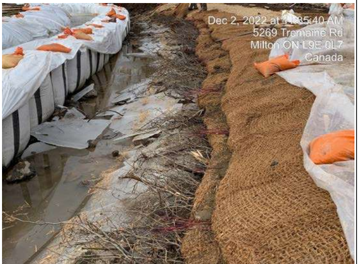
Pond 2 Area Enhancement - Installation of material for Riffle
