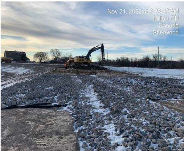
Pond 1- Excavation of material for Emergency Spillway
