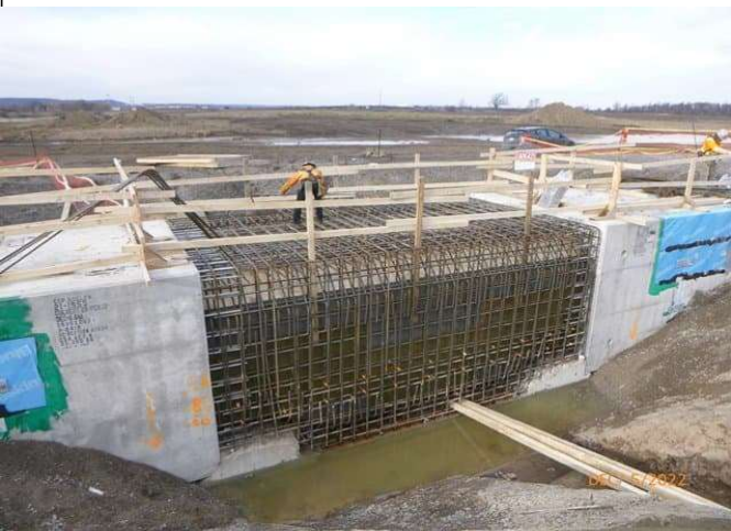
Box Culvert 2B - Reinforcement placement at cast in place section
