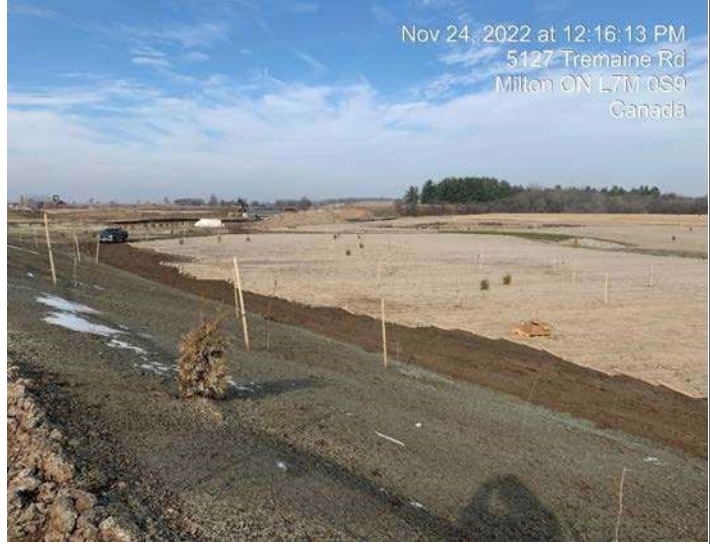
Indian Creek Area - Installation of Jute Matting along topsoiled areas
