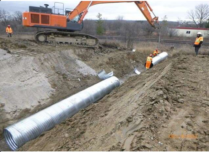
East Track Diversion - 900mm csp culvert crossing install at Stn. 65+325
