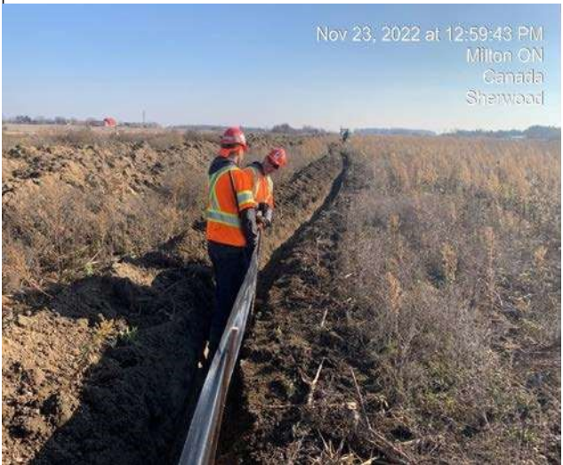
East Track Diversion - Installation of silt fencing
