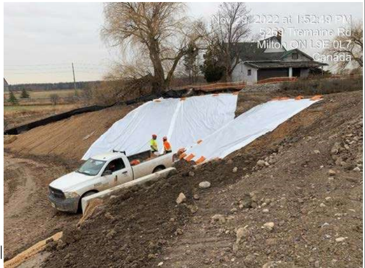
Pond 2 Area - Protection cover of slopes with poly tarps.
