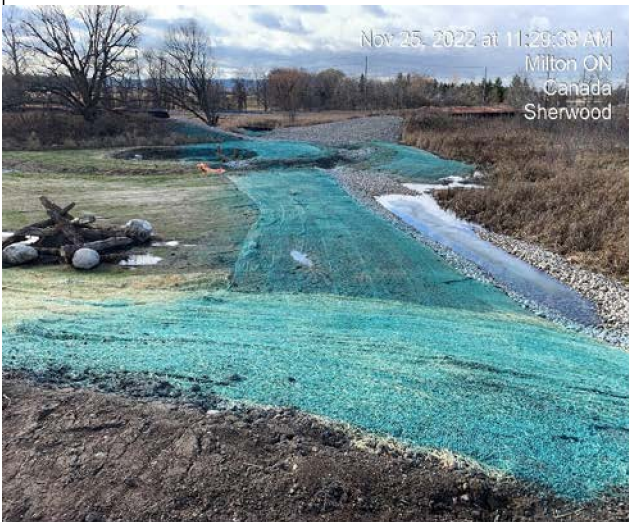
Pond 1/Tributary A - Hydroseed topsoiled areas
