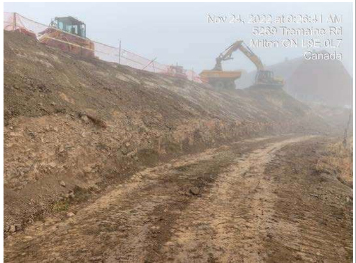
Pond 2 Area - Excavation of material for slope grading along embankment
