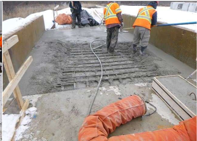
Trib. A - Concrete placement for cast in place box culvert 2A
