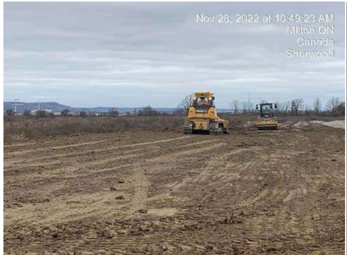
East Track Diversion - Grading of cut/fill material for track diversion
