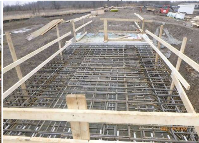
Box Culvert 2A - Reinforcement placement at cast in place section
