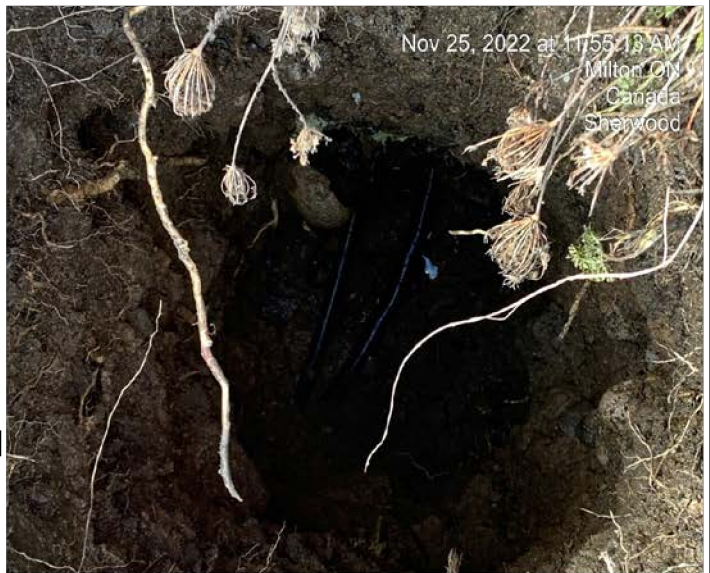
North Track Crossing - Hi-Rail vac truck locating signal cables along ROW
