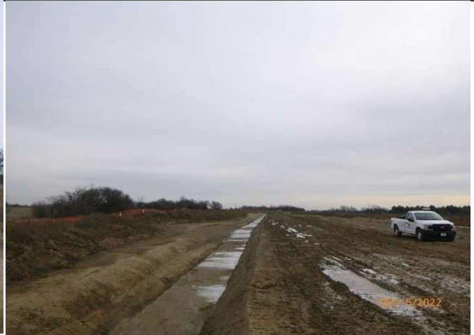
East Track Diversion - Grading/shaping ditches facing South to Culvert 3
