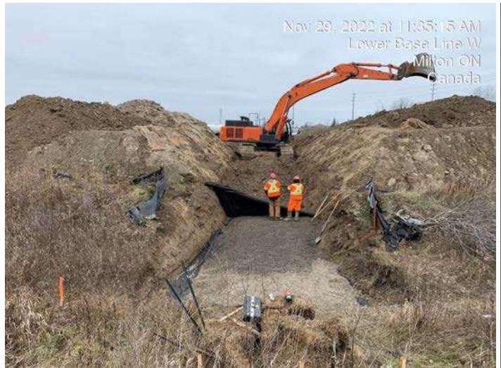
East Track Diversion - Excavation and bedding installation for storm sewer
