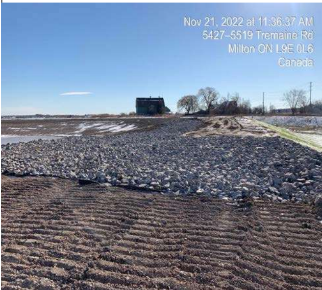
Pond 1- Excavation of material for Emergency Spillway
