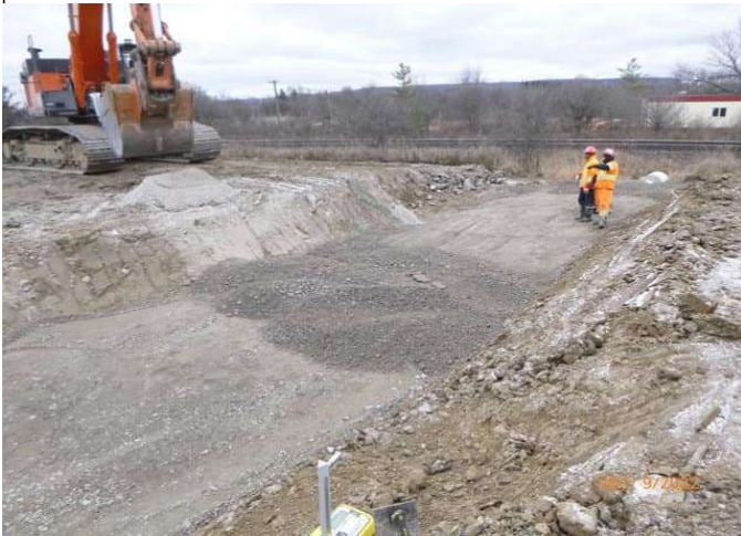
East Track Diversion - Backfill/Compacting culvert crossing at Stn. 65+325
