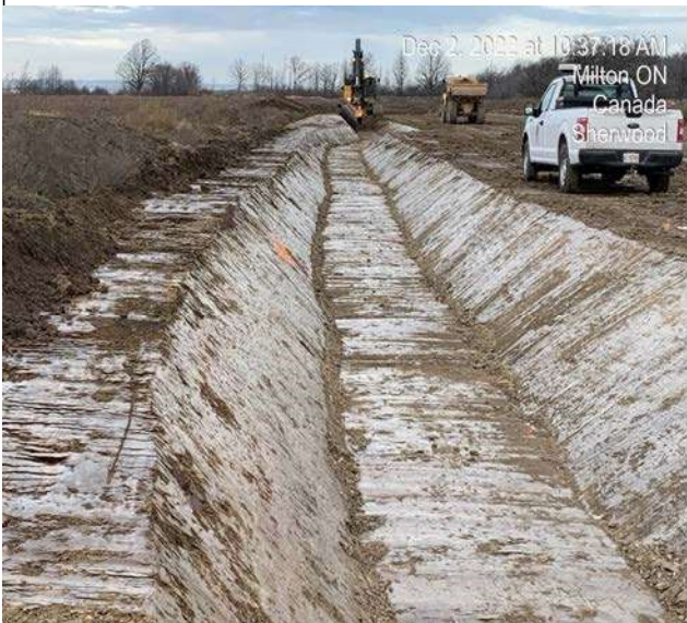
East Track Diversion - Excavation of west side ditch cut to fill
