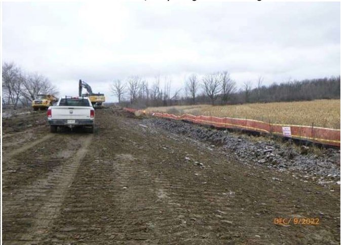
East Track Diversion - Grading track shoulder slope South of Trib. A
