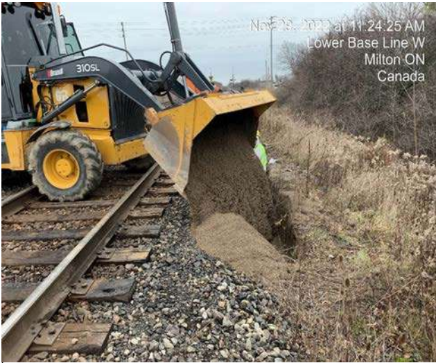
Lower Baseline Area - Backfill trench at culvert crossing location
