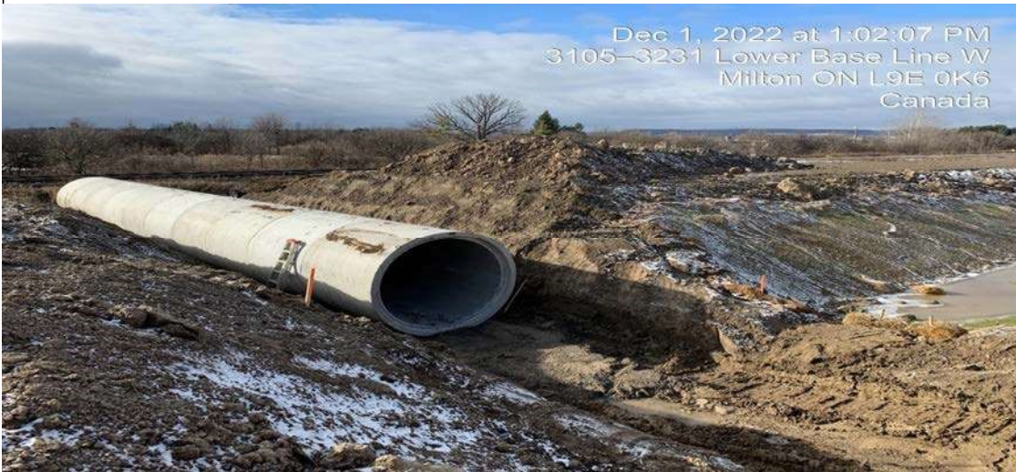
East Track Diversion - Installation of 2400mm concrete storm sewer
