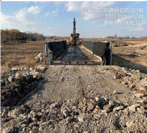
Indian Creek - Begin dismantle south approach sections at bridge
