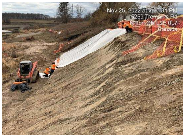
Pond 2 Area Creek Diversion- Install poly tarp along completed slope.
