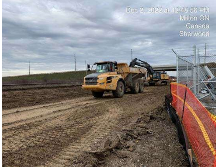
North Crossing Area - Continue striping and grading along ROW
