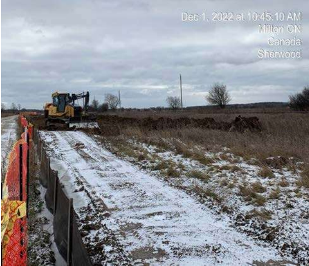
East Track Diversion - Grading of cut/fill material for track diversion
