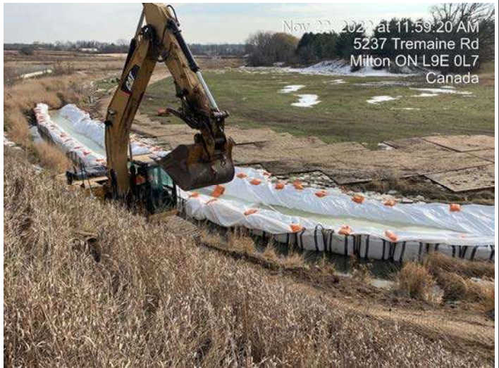
Pond 2 Area - Excavation of material for riffle installation as per design
