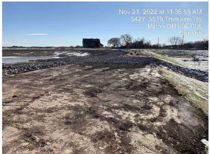
Pond 1- Excavation of material for Emergency Spillway
