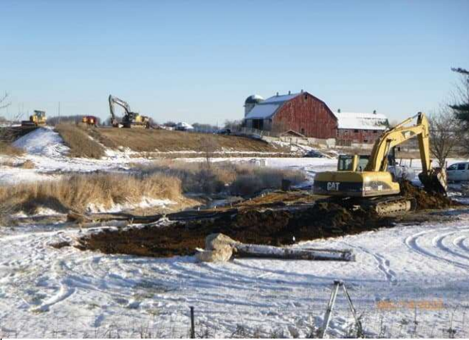
Indian Creek - Excavation for Riparian Wetland pond at enhancement section
