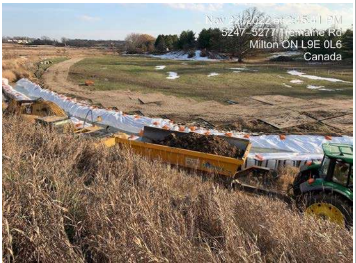
Pond 2 Area - Excavation of material for riffle installation as per design
