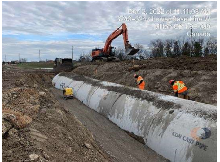
East Track Diversion - Backfill and compact 2400mm concrete storm sewer
