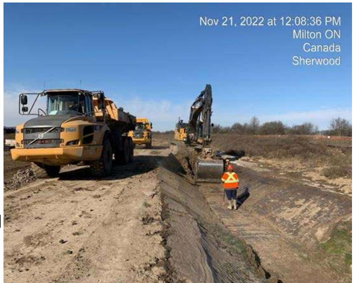
East Track Diversion - Excavation and grading for track diversion grading
