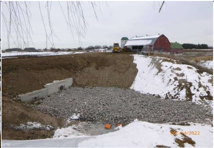
SWM Pond #2 - Grading outlet channel at Headwall P2D
