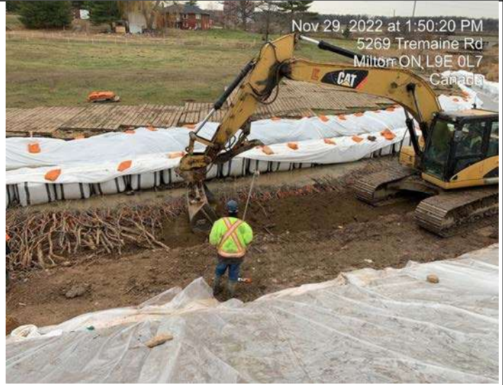
Pond 2 Area Enhancement - Installation of material for Riffle
