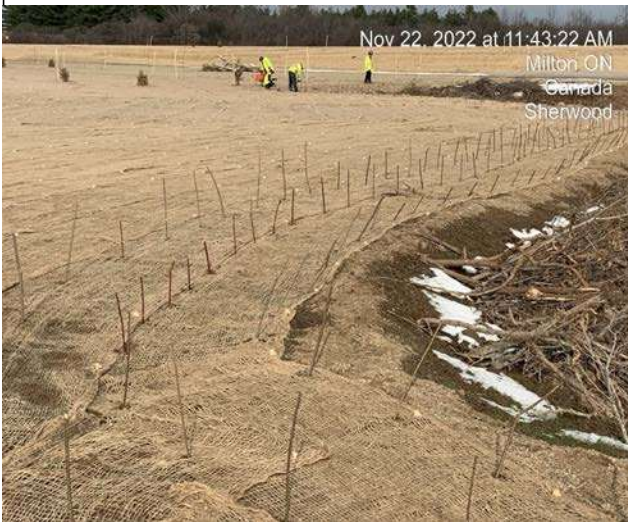
Indian Creek - C.L. install live stakes along Riparian Wetland areas
