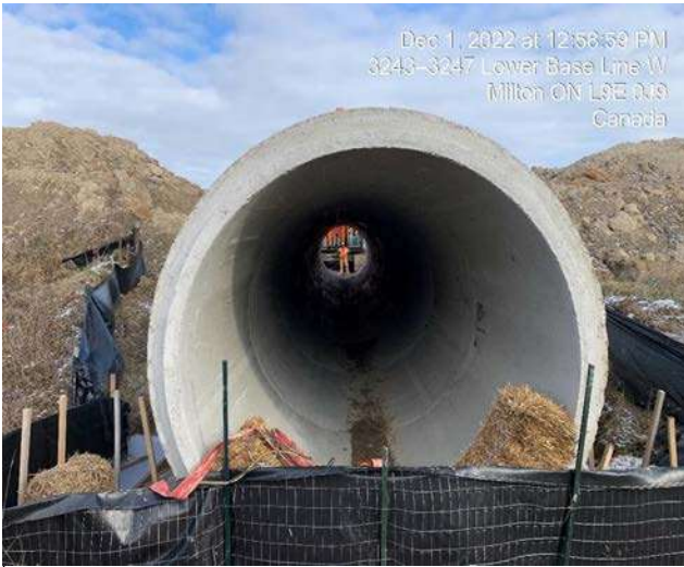
East Track Diversion - Installation of 2400mm concrete storm sewer
