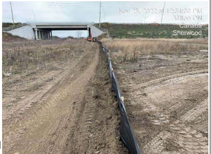
North Crossing Area - Installation of silt fencing along ROW as per design.
