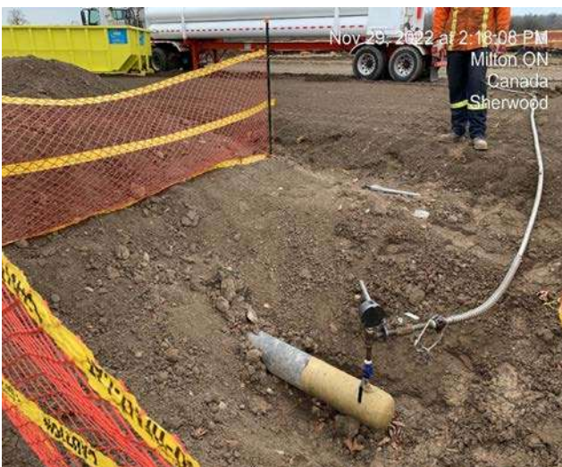
Sun Canadian - Pumping of Nitrogen gas into abandoned pipeline
