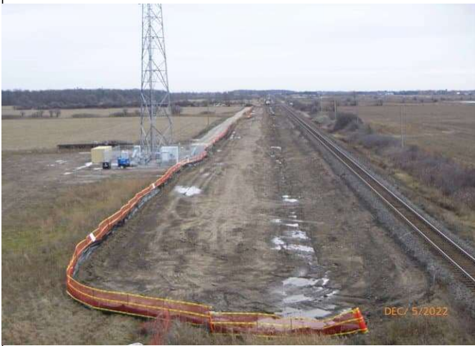
Track Realignment - Stripped topsoil for track realignment South of Britannia bridge
