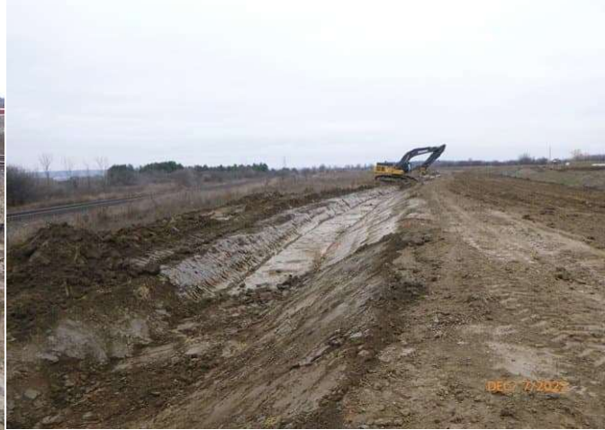
East Track Diversion - Grading/shaping West ditch North of Culvert 3
