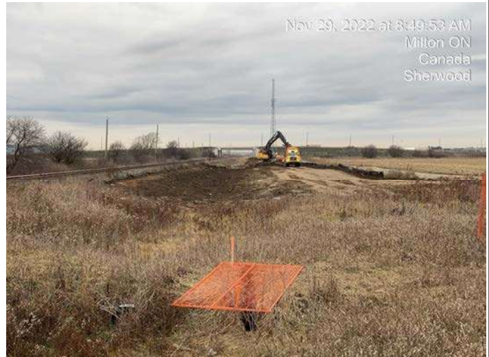
North Crossing Area - Continue striping and grading along ROW
