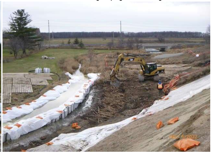
Indian Creek - Wooden Toe Protection construction along enhancement areas
