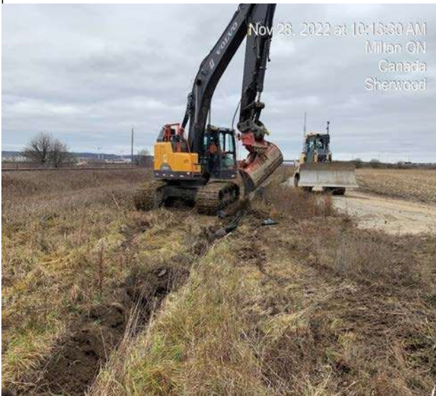
North Crossing Area - Begin striping and grading along ROW
