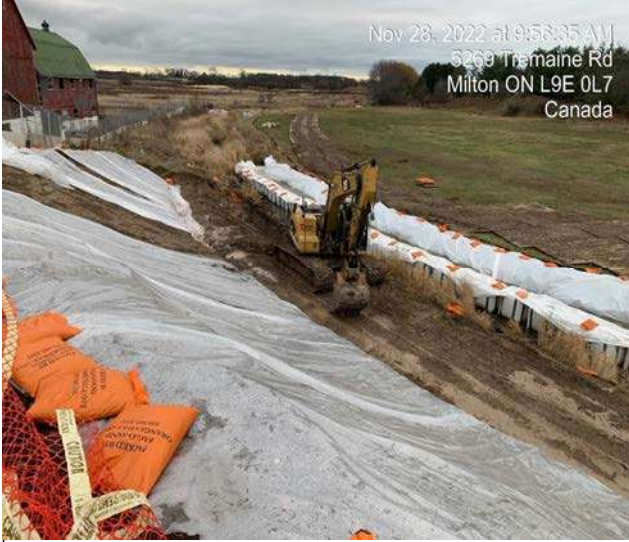
Pond 2 Area Enhancement - Excavation of material for Riffle installation
