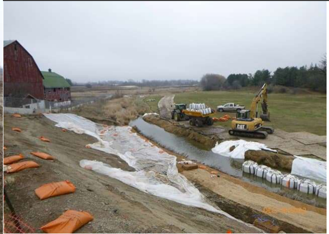
Indian Creek - Cofferdam removal along completed enhancement section
