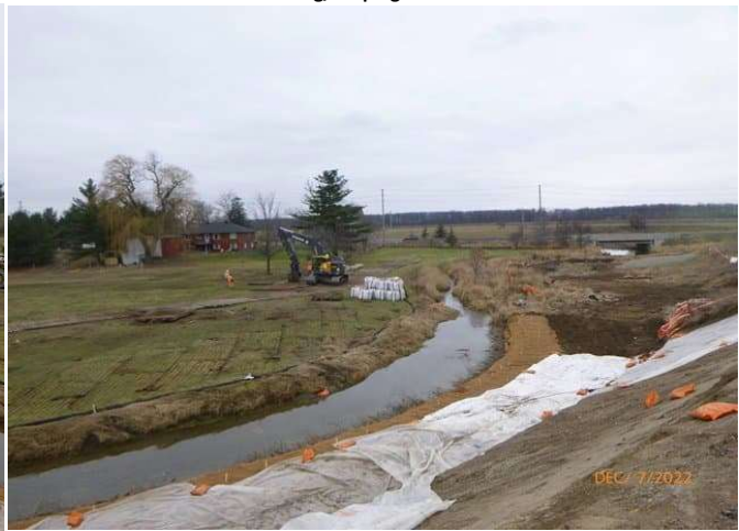
Indian Creek - Relocate matting for next cofferdam enhancement section
