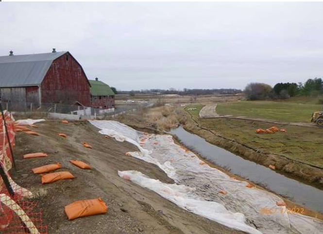
Indian Creek - Removed cofferdam at completed enhancement section
