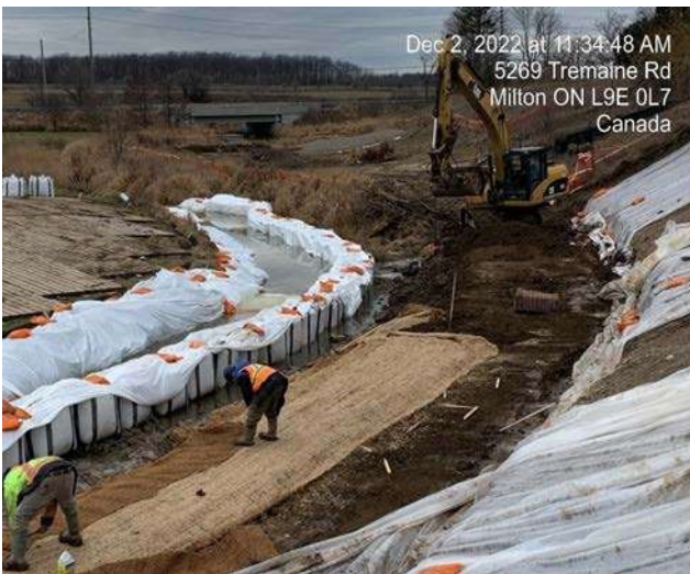
Pond 2 Area Enhancement - Installation of material for Riffle
