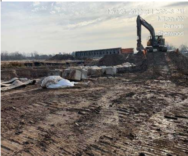
Indian Creek - Removals of north side bridge abutment
