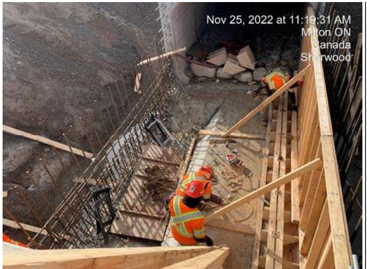
Trib A Box Culvert - Installation of forms and bracing for Cast in Place section
