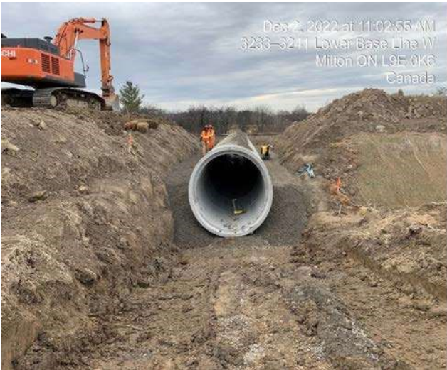
East Track Diversion - Backfill and compact 2400mm concrete storm sewer
