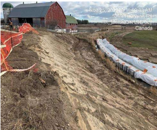
Pond 2 Area Creek Diversion- Excavation of material for slope grading
