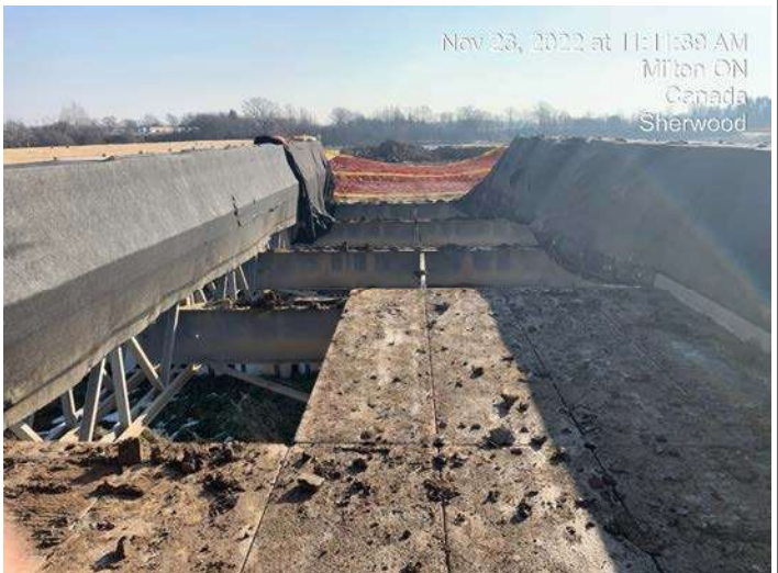
Indian Creek - Dismantle and remove bridge decking
