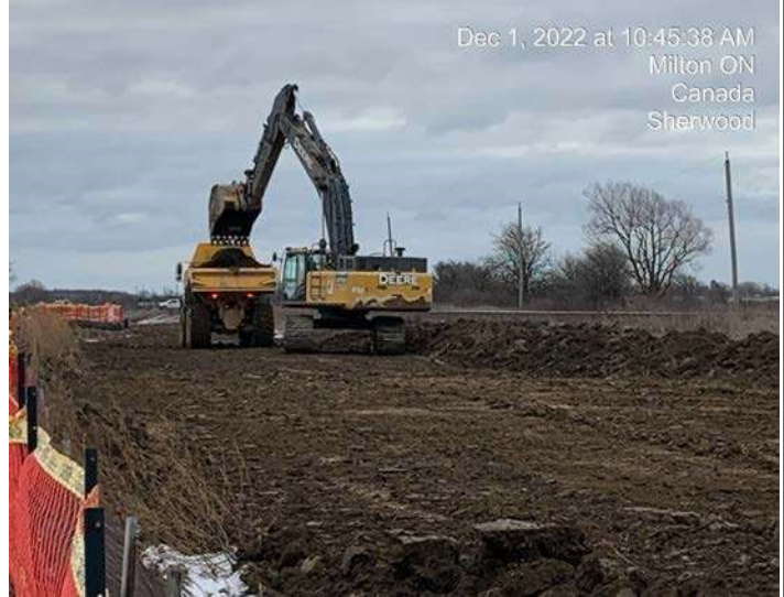
East Track Diversion - Grading of cut/fill material for track diversion
