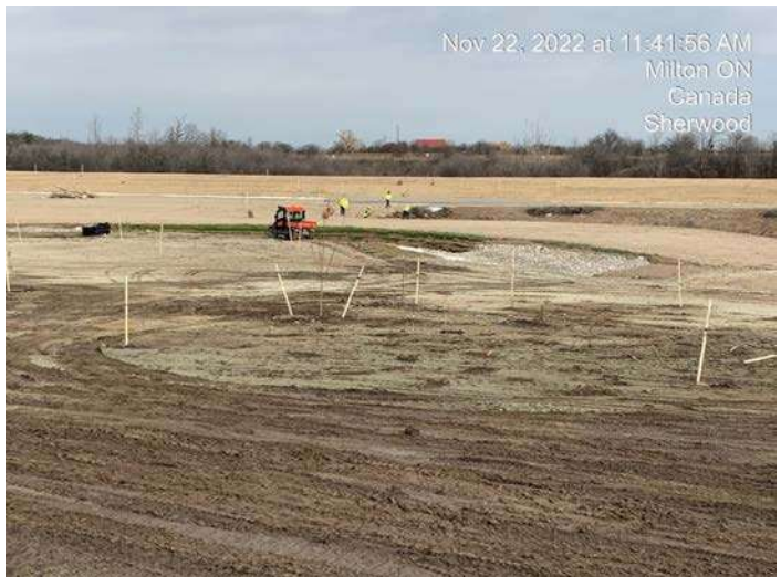
Indian Creek - C.L. install stake supports for trees and bushes
