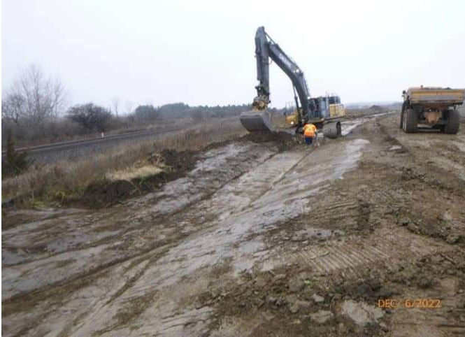
East Track Diversion - Grading/shaping West ditch North of Culvert 3
