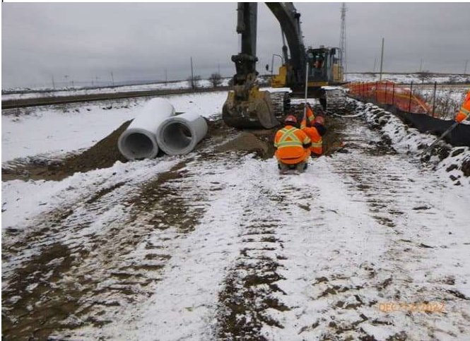
Track Realignment Sewer - 750mm conc. Storm sewer install at Stn. 62+650
