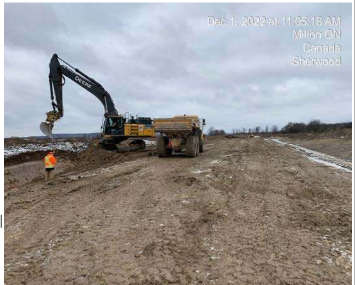
East Track Diversion - Excavation of west side ditch cut to fill
