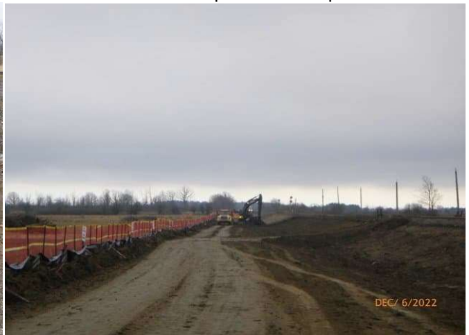
Track Realignment - Stripping topsoil for track realignment South of Sun Canadian track crossing
