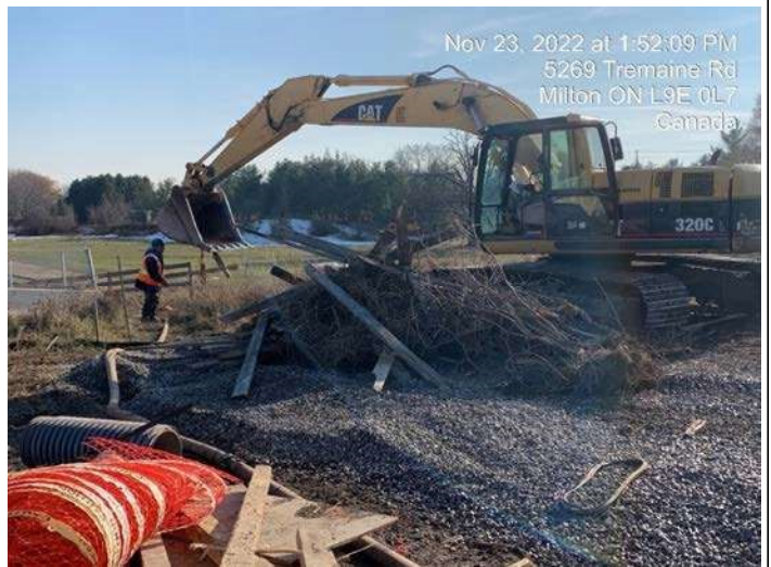
Pond 2 Area - Removal of existing farm fence for slope grading
