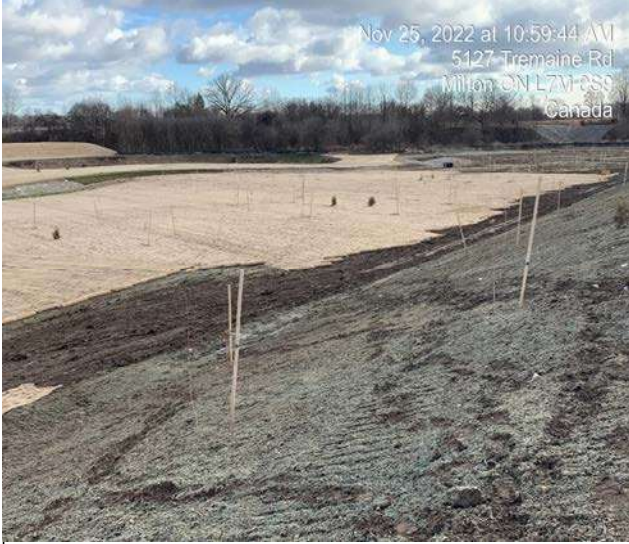
Indian Creek Area - Installation of Jute Matting along topsoiled areas
