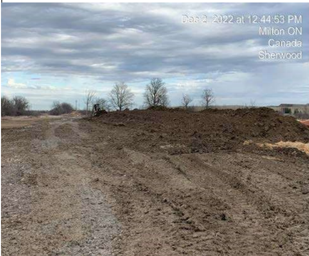
North Crossing Area - Grading of stockpiled topsoil from stripping area.
