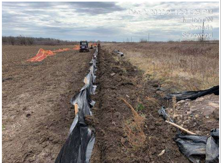
North Crossing Area - Installation of silt fencing south of north crossing
