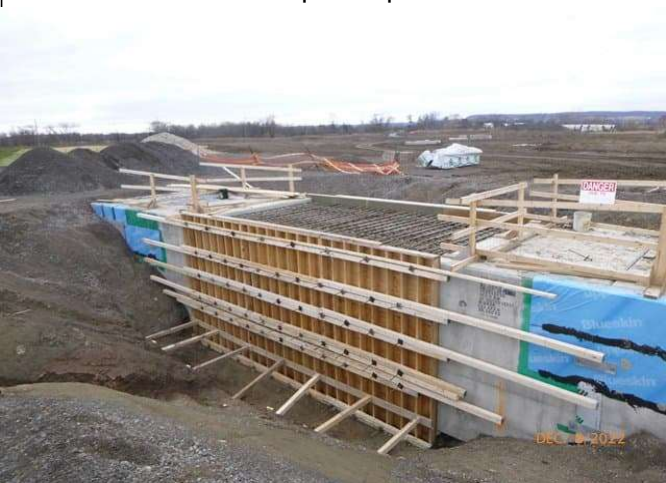
Box Culvert 2B - Installed exterior forms for cast in place section
