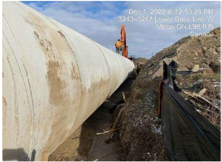
East Track Diversion - Installation of 2400mm concrete storm sewer
