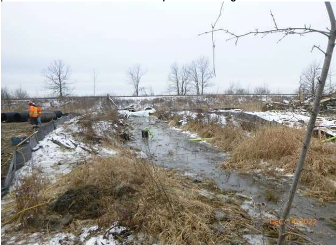
Trib. A - Fish rescue and dewatering creek section at prop. Track realignment
