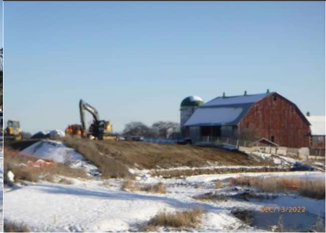
Indian Creek/SWM Pond 2 - Shape berm along enhancement area
