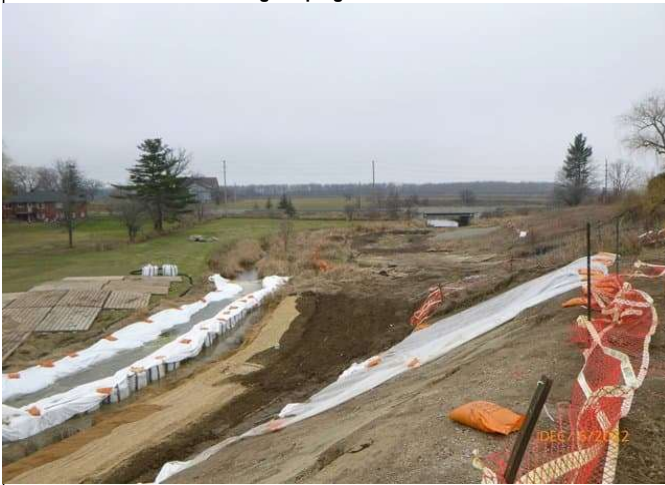
Indian Creek - Completed Wooden Toe Protection enhancement section
