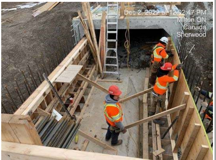
Trib A Cast-in-Place - Installation of interior forms for middle box culvert section
