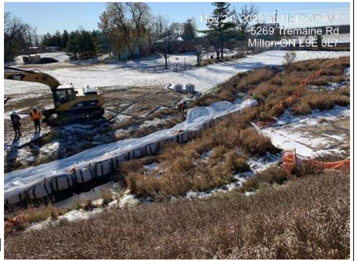
Pond 2 Area - Installation of poly tarps and sand bags for coffer dam
