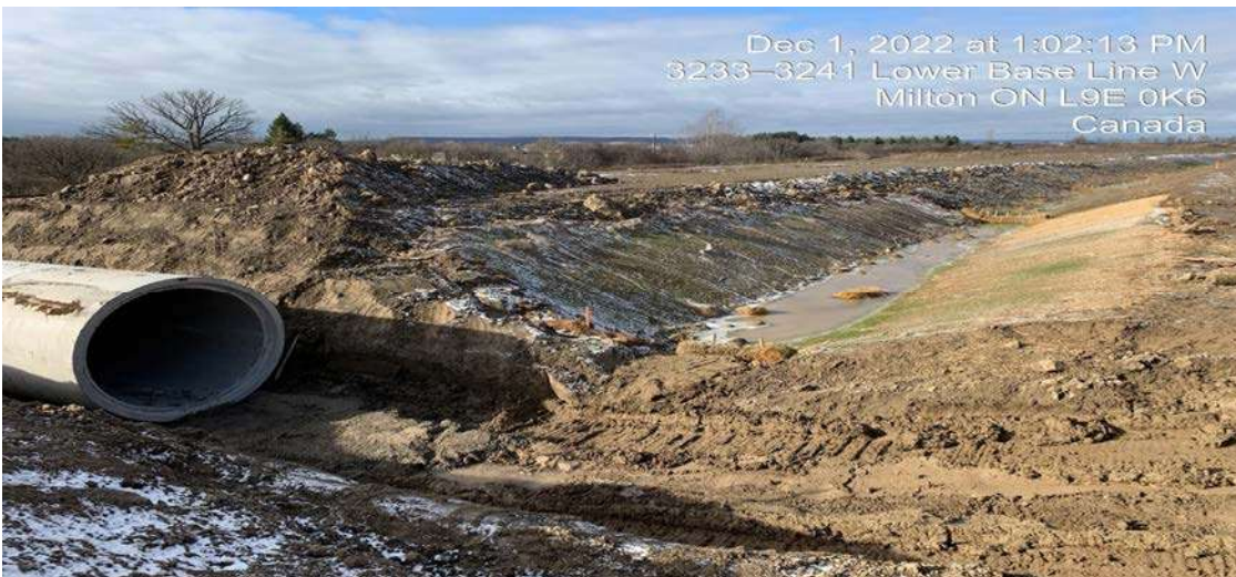
East Track Diversion - Installation of 2400mm concrete storm sewer
