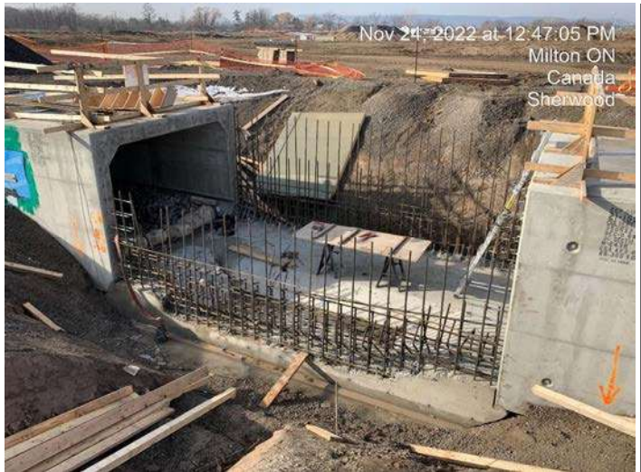
Trib A Box Culvert - Continue works on Cast in Place section
