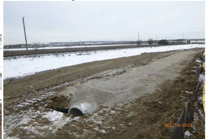
SWM Pond #2 - Grading outlet channel at Headwall P2D
