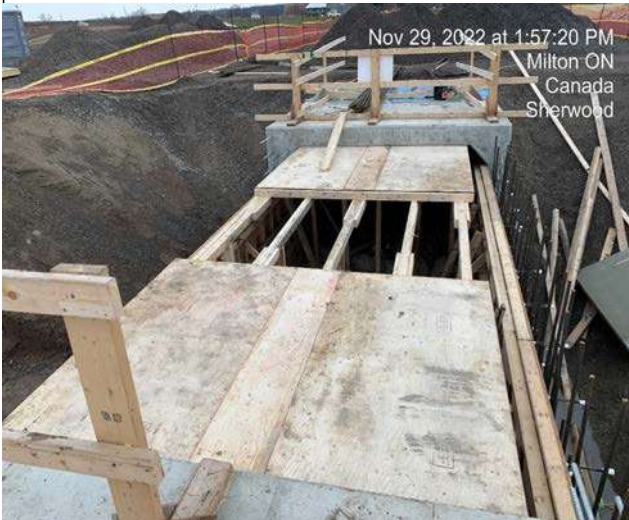
Trib A Cast-in-Place - Installation of interior forms for box culvert section
