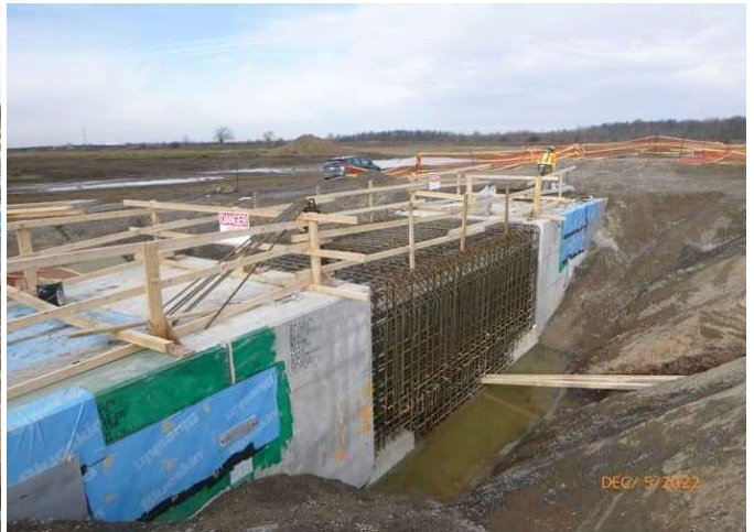
Box Culvert 2B - Reinforcement placement at cast in place section
