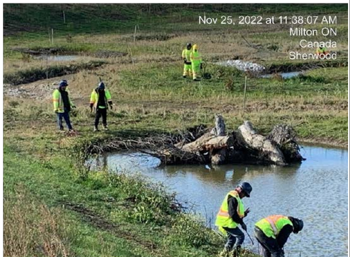
Tributary A - Install live stake plantings along creek diversion.
