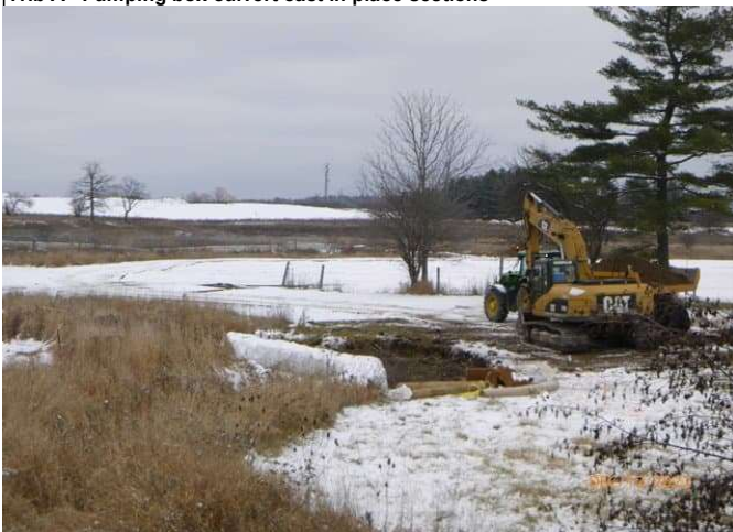
Indian Creek - Excavation for wooden toe debris enhancement section
