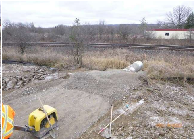
East Track Diversion - Backfill/Compacting culvert crossing at Stn. 65+325
