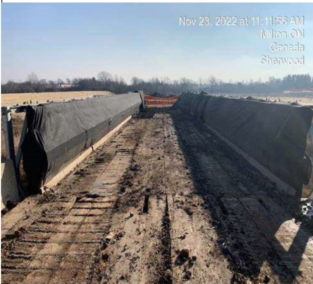
Indian Creek - Dismantle and remove bridge decking
