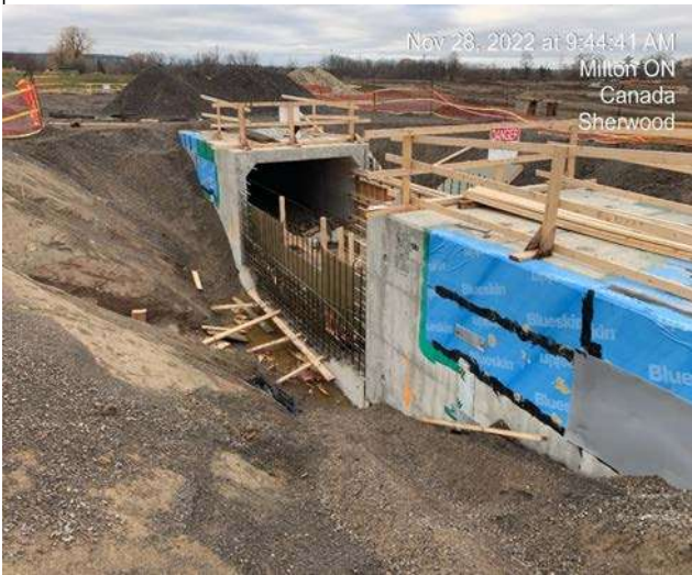
Trib A Cast-in-Place Culvert - Forming of inner walls for box culvert
