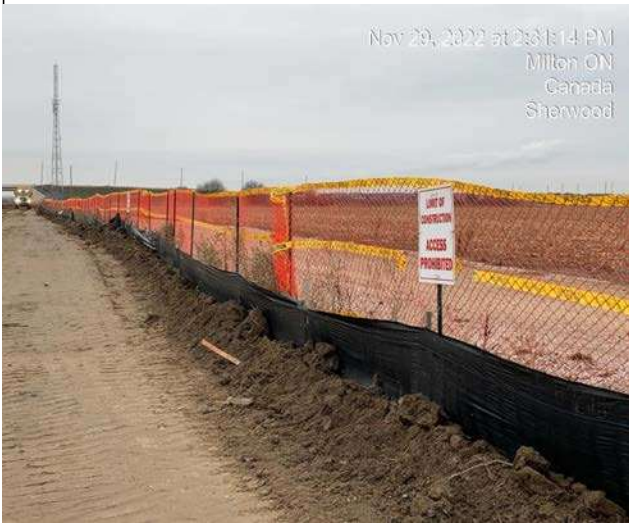
North Crossing Area - Installation of construction fencing along the ROW
