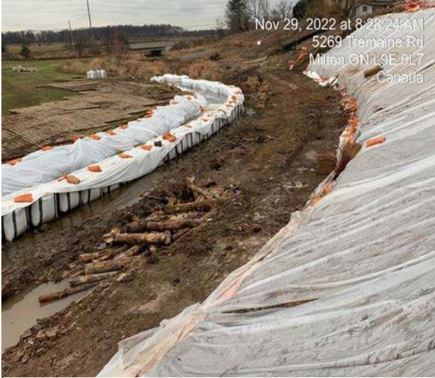
Pond 2 Area Enhancement - Installation of material for Riffle
