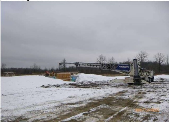
Trib A - Pumping box culvert cast in place sections
