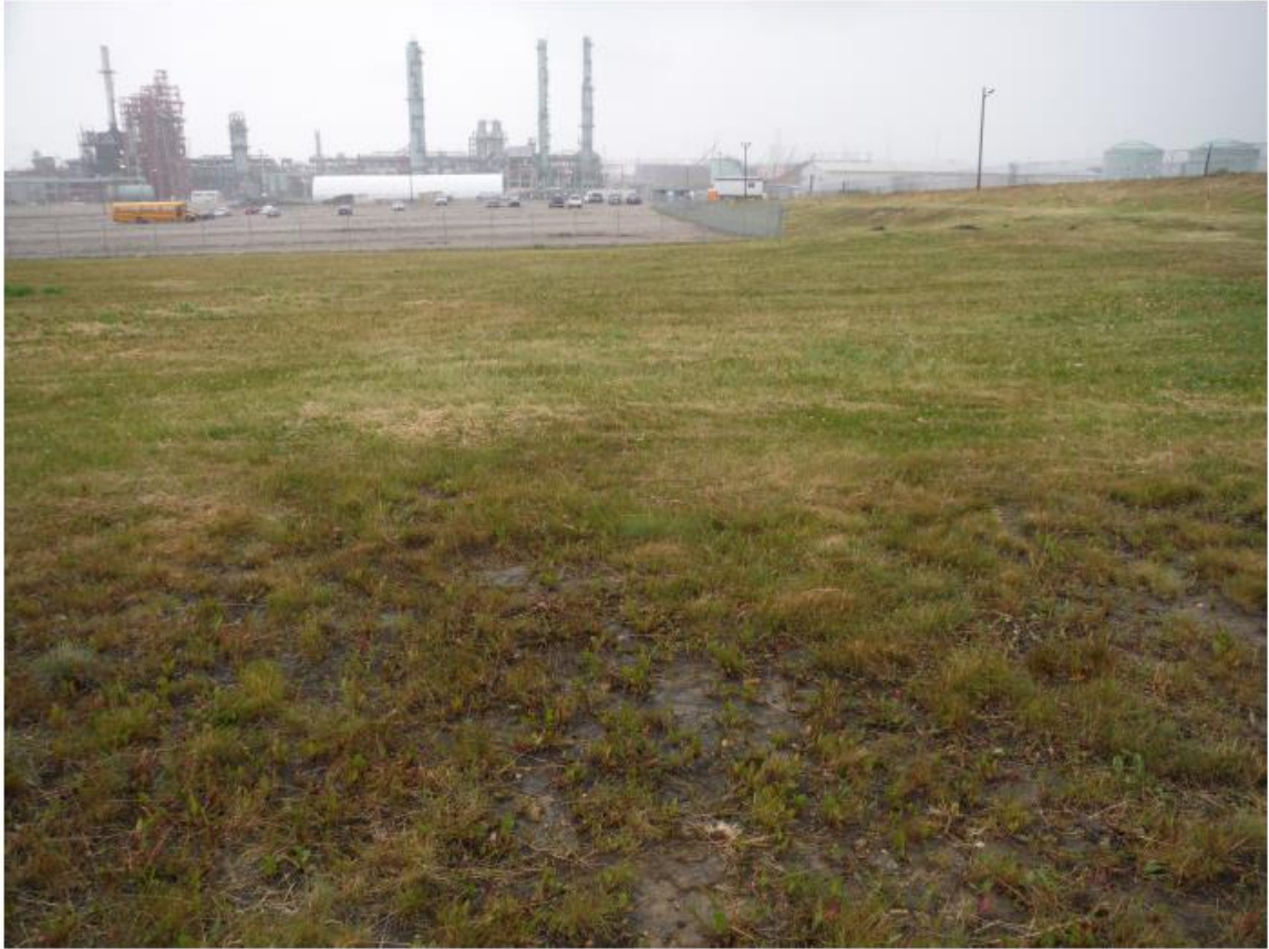
Figure 7 - BTT Location Facing North
