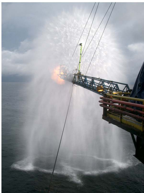
Photo 1 Boom Cooling System (Source: Optima 2014)
