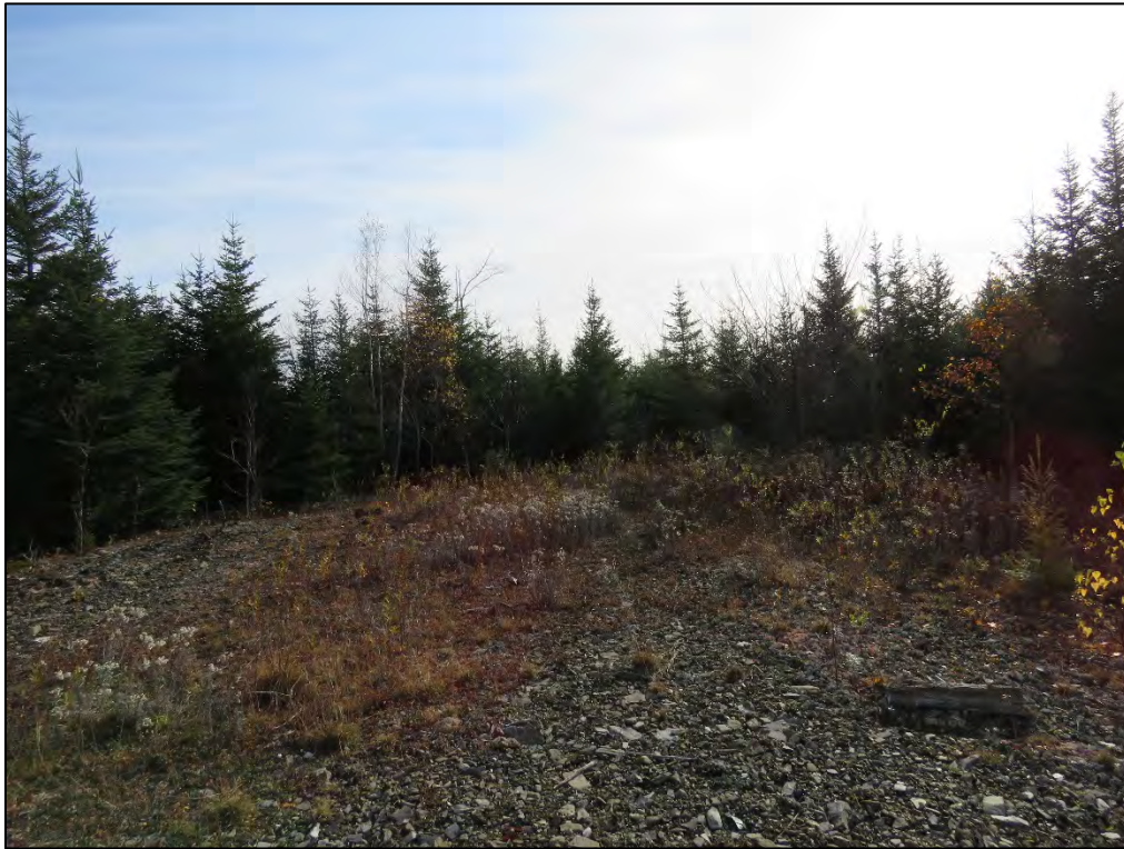
Plate 3: Portion of Area 2 levelled and covered with rock/gravel. Facing southeast; October 26, 2020.
